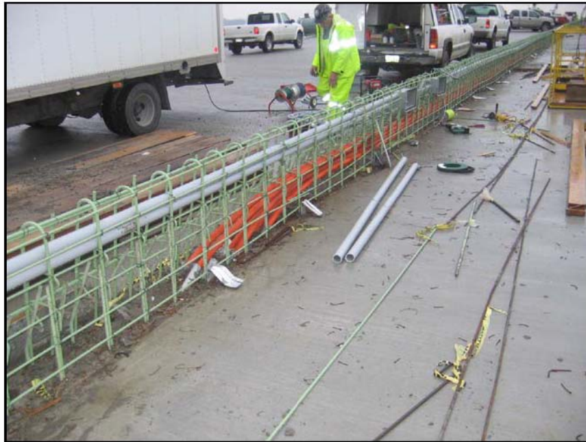
Figure 5 - Example of Conduit on Bridge Structure
