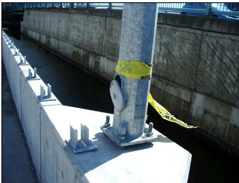
Figure 4 - Example Foundation on Bridge Structure
