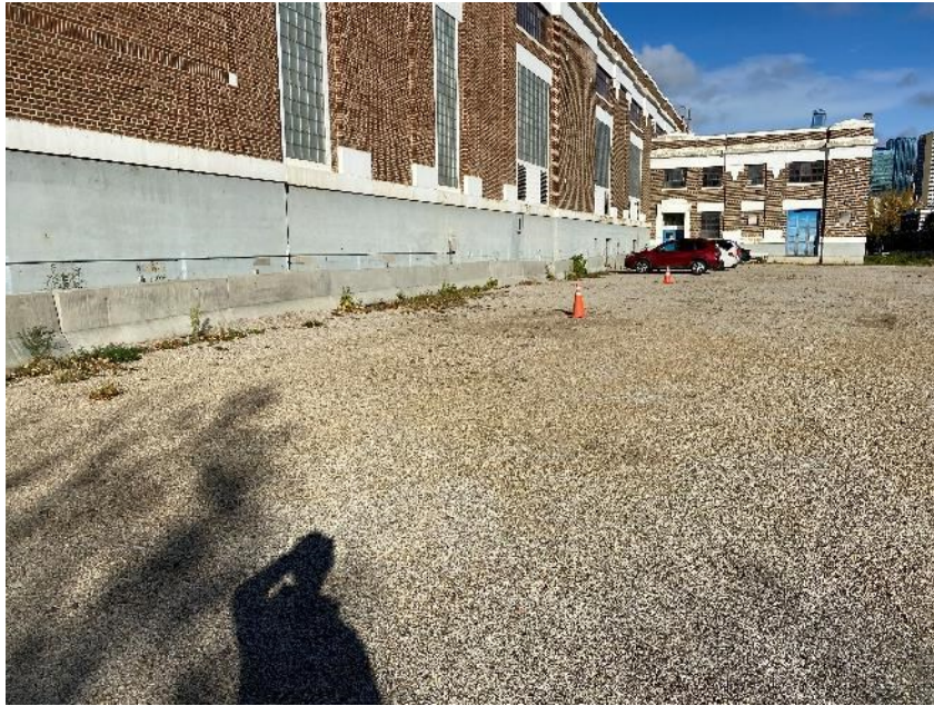
Above: Parking lot local low spots and negative drainage
