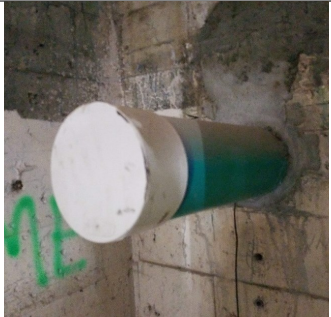
Above: 150mm Sanitary Connection North
