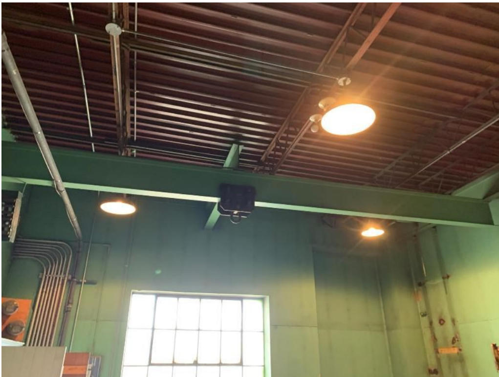
Above: Switch House – Roof Structure
