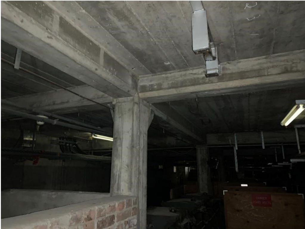
Above: Switch House – Basement
