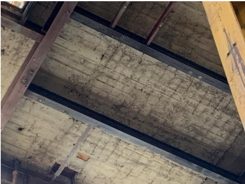
Above: Boiler Hall – Concrete on Mezzanine Structure
