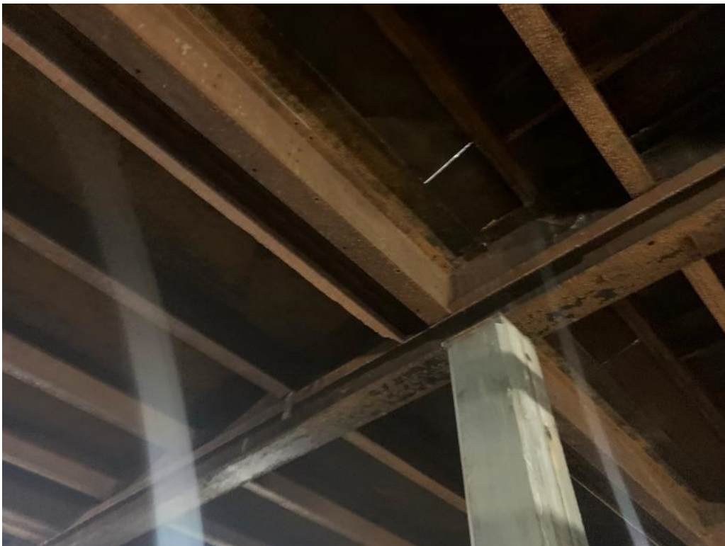
Above: Boiler Hall – Basement Structure
