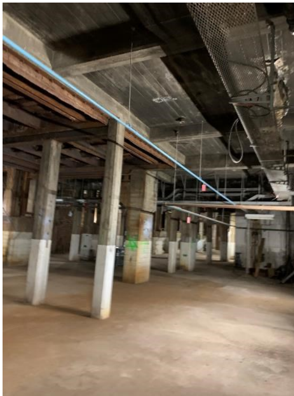
Above: Boiler Hall- Basement Structure
