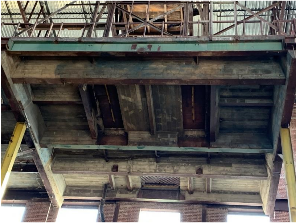
Above: Boiler Hall – Mezzanine Structure
