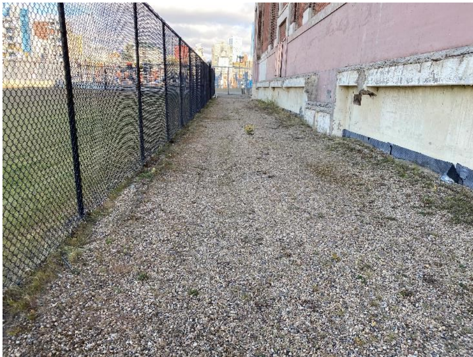
Above: Low slope away from the Low Pressure Plant West Elevation
