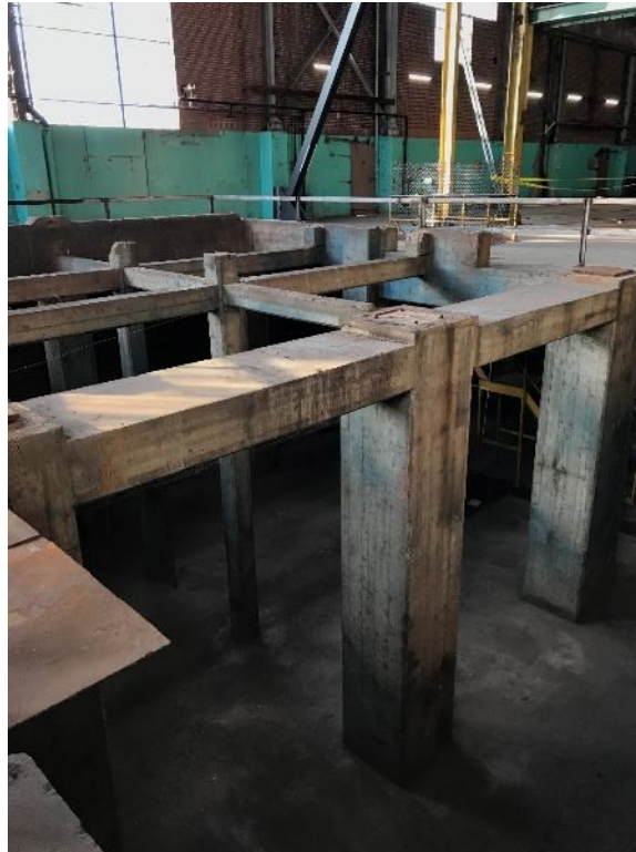
Above: Boiler Hall – Main floor Structure
