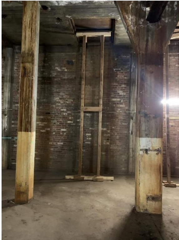
Above: Boiler Hall - Support Structure Typical for Openings
