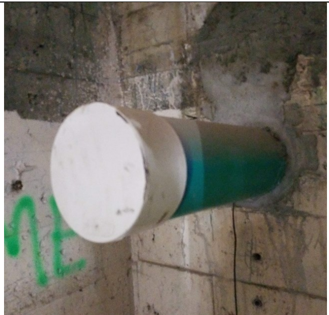
Above: 150mm Sanitary Connection North
