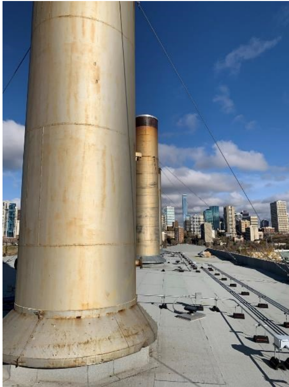
Above: Boiler Hall – Smokestacks on Roof
