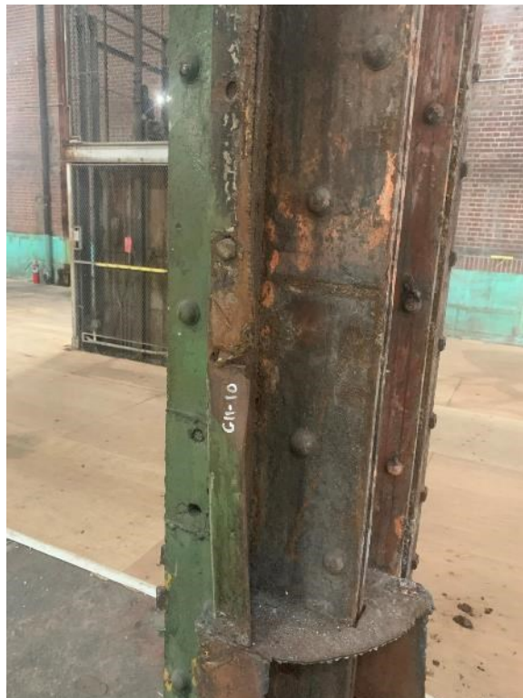
Above: Boiler Hall- Modified Structure
