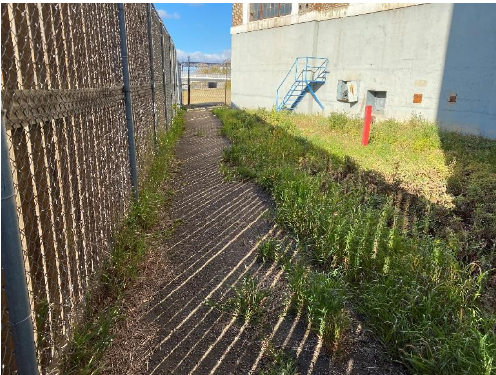
Above: Negative drainage and flow restriction cause by path
