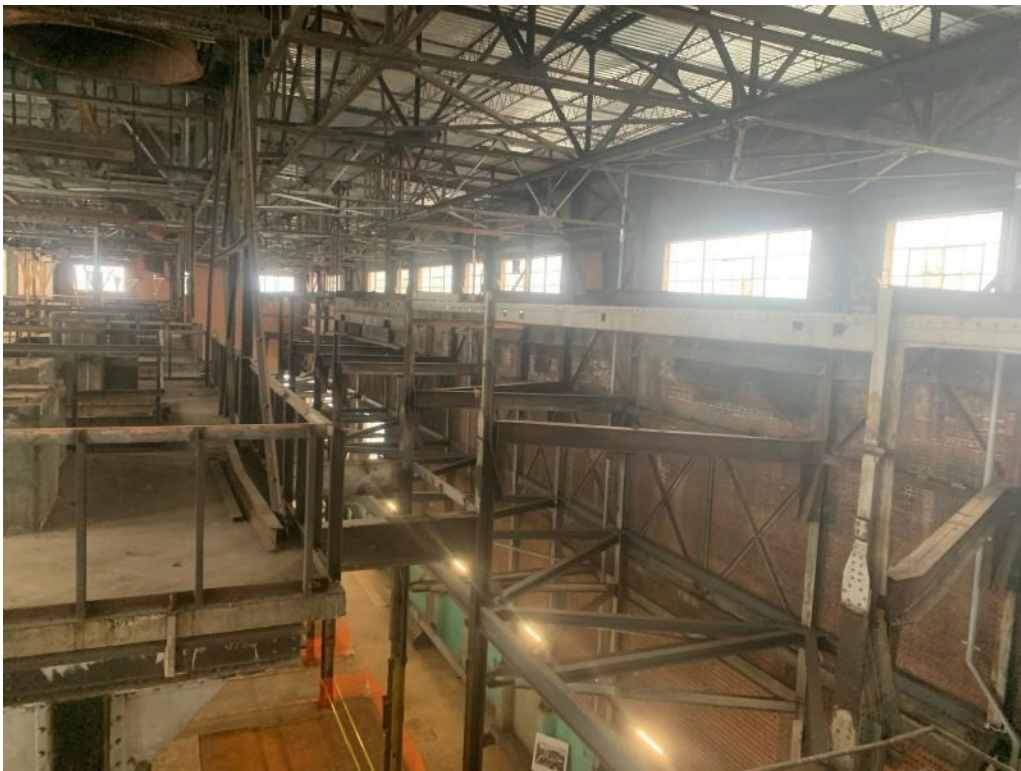
Above: Boiler Hall – Roof Structure
