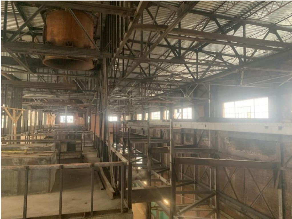
Above: Boiler Hall – Roof and Mezzanine Structure
