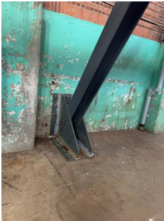
Above: Boiler Hall – Reinforcement of West Wall
