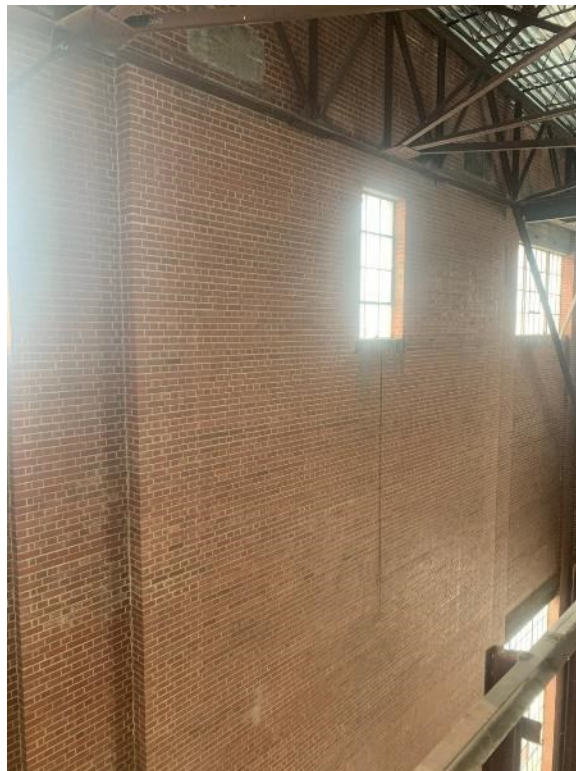
Above: Boiler Hall – Exterior Brick Wall
