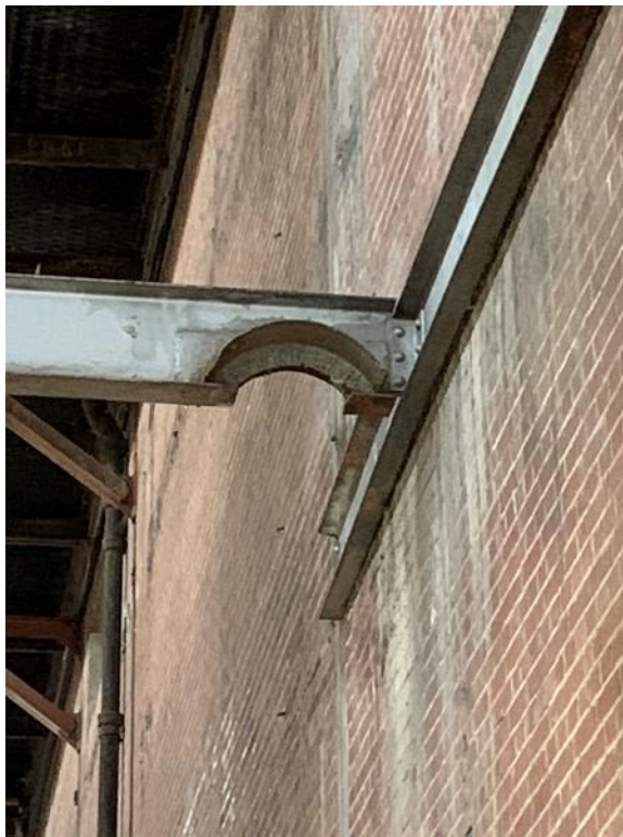
Above: Boiler Hall – Typical Modified Structure
