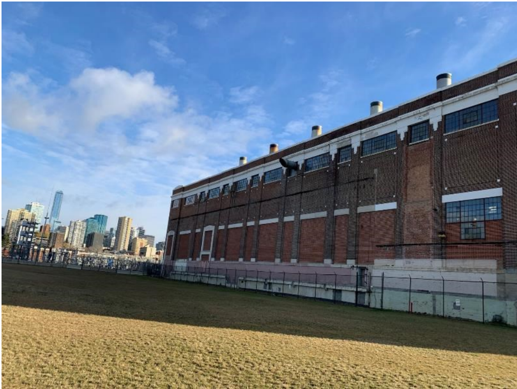
Above: West Wall of Boiler Hall
