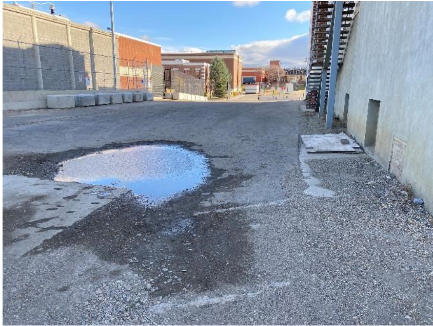
Above: Water pooling in settled asphalt area north of the Low Pressure Plant
