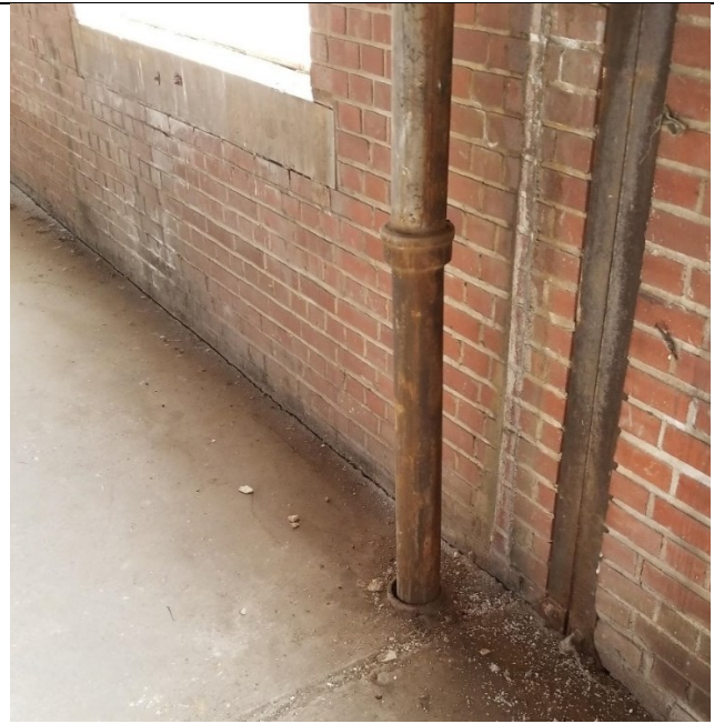
Above: Cast iron rainwater leader, Boiler Hall
