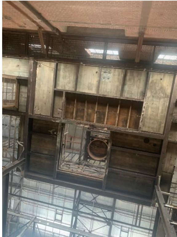
Above: Boiler Hall – Smokestack structure
