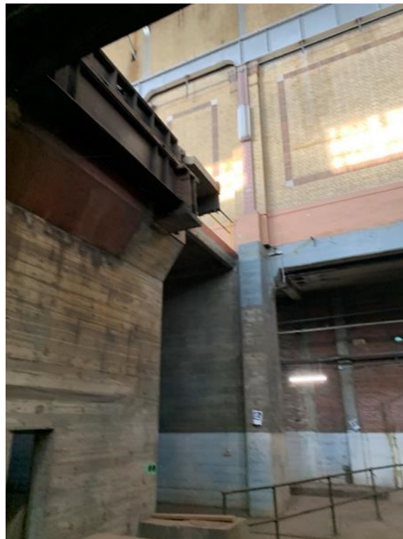
Above: Turbine – Basement Structure
