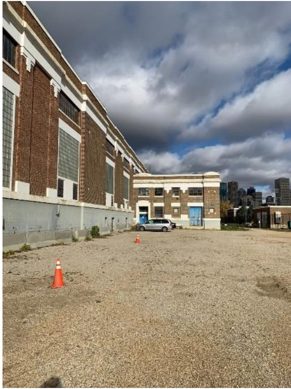
Above: Turbine/Switch house
