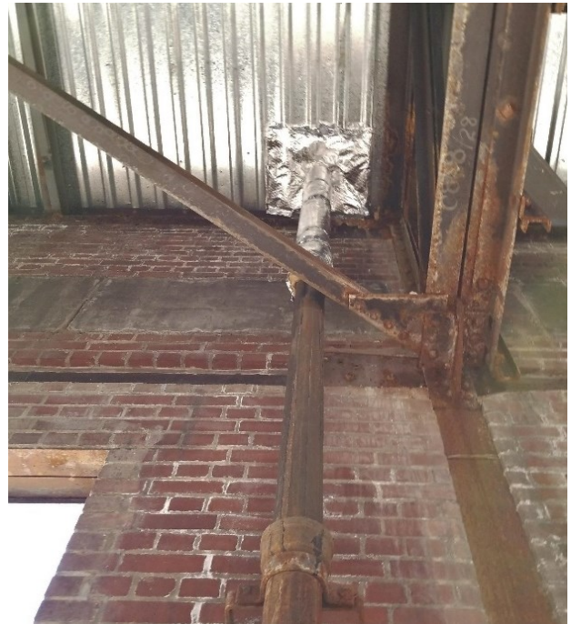
Above: New roof drain and connection to RWL (boiler hall)
