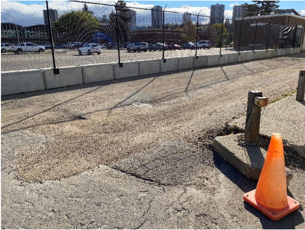
Above: Storm catch basin east of the Switch House
