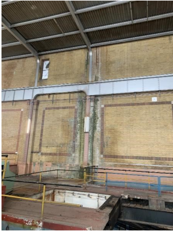
Above: Turbine –Shared Wall with Boiler Hall
