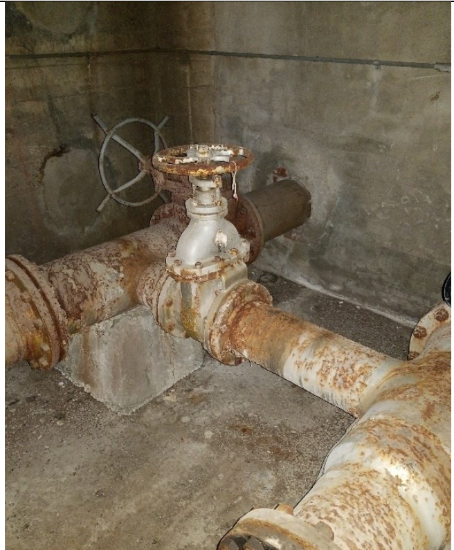
Above: 300mm steel gas piping
