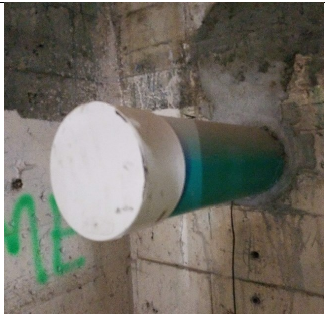
Above: 150mm Sanitary Connection North
