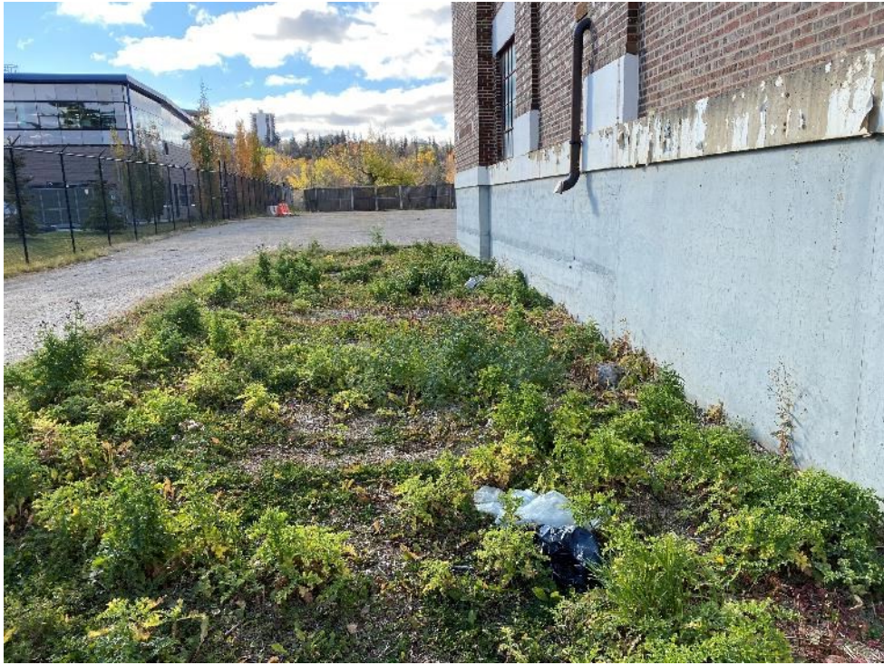
Above: Landscaped area east of the Switch House
