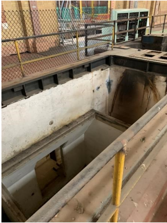
Above: Turbine –Main Floor Structure
