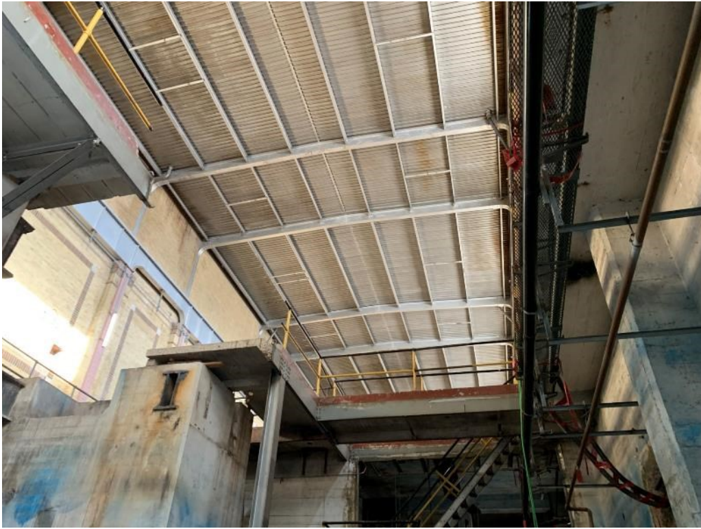
Above: Turbine – Photo from basement
