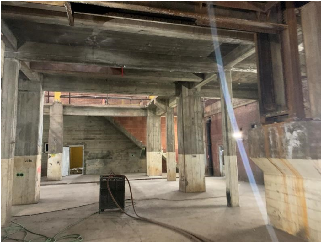
Above: Turbine –Basement Structure
