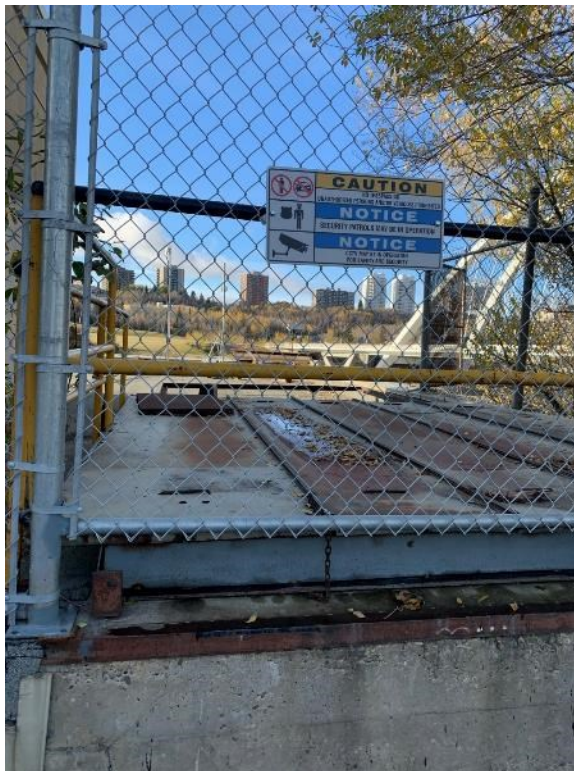
Above: PH2 – Main Roof Structure from Exterior
