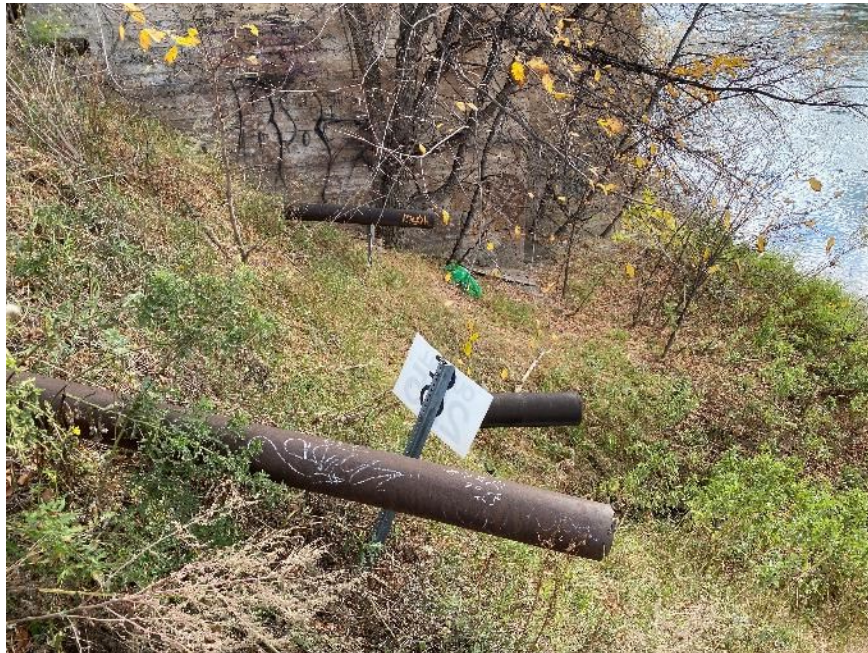
Above: Outfalls possibly from building storm leaders west of Pump House 2
