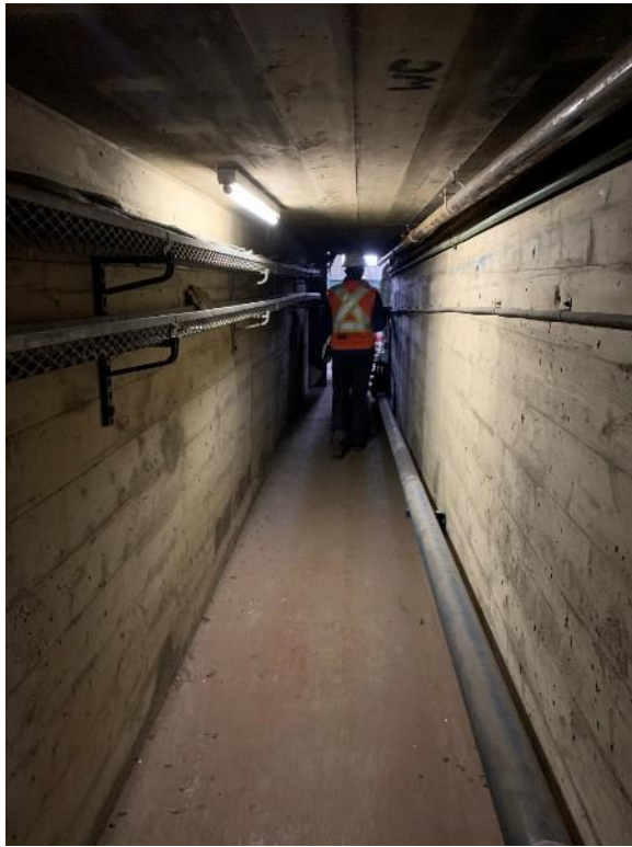
Above: PH1- Tunnel from Turbine Hall
