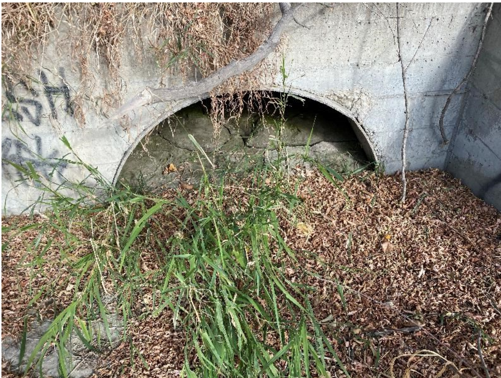
Above: Abandoned outfall piping from building
