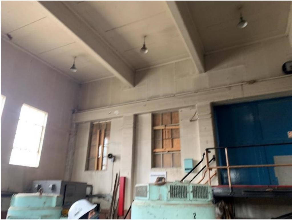
Above: PH1 – Roof Structure
