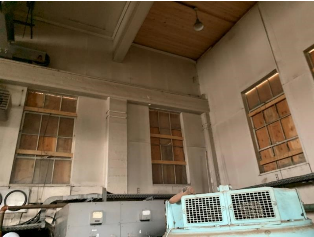
Above: PH1 - Roof Structure
