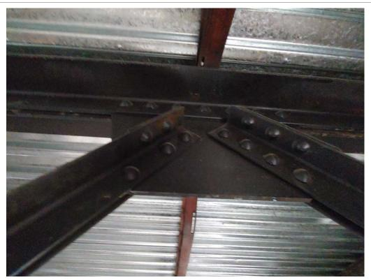
Photo 31: Roof - Truss bolting
