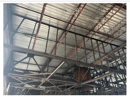
Photo 29: Roof – Joists and miscellaneous framing.
