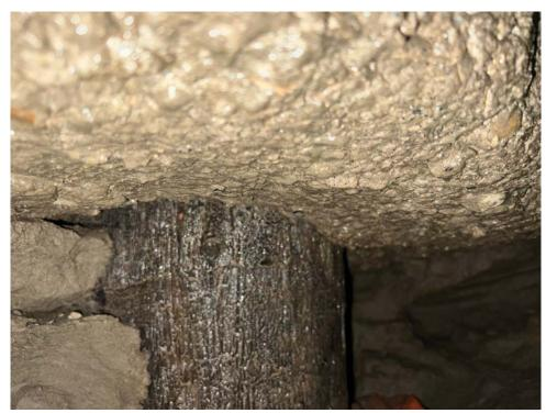
Figure 8: Wood Pile Surface
