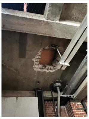
Photo 6: 2nd Floor – Opening to infill
