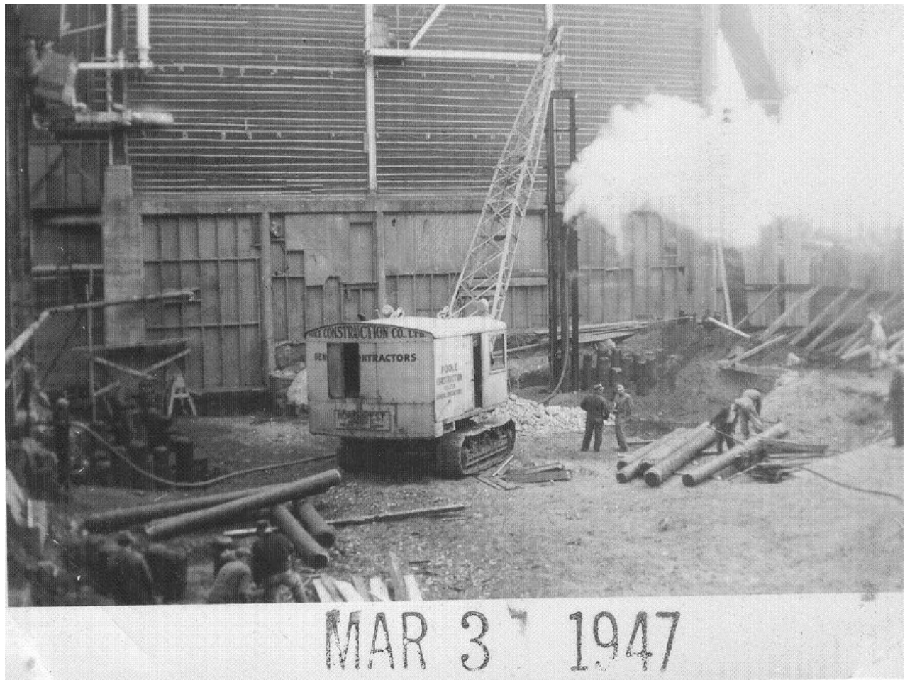
Figure 10: Poole Construction Limited (PCL) using crane to drive piles in the 1947 power plant addition. (Source: EPHF)
