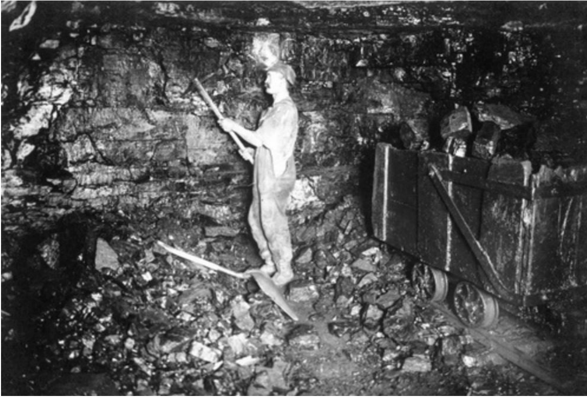
Figure 126: Coal mining by pick, note the coal truck on rail behind this worker. The working conditions were dangerous and difficult. (Source: Humberstone Fonds. CEA, EB-39-7)
