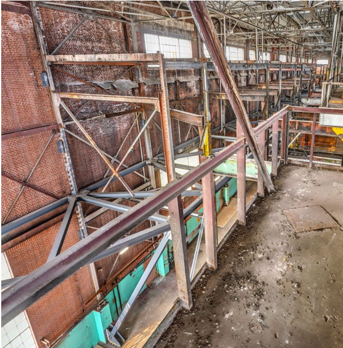
Figure 15: Gray steel below is modern reinforcement all other riveted steel is original. (Source: Cloud360, 2020)
