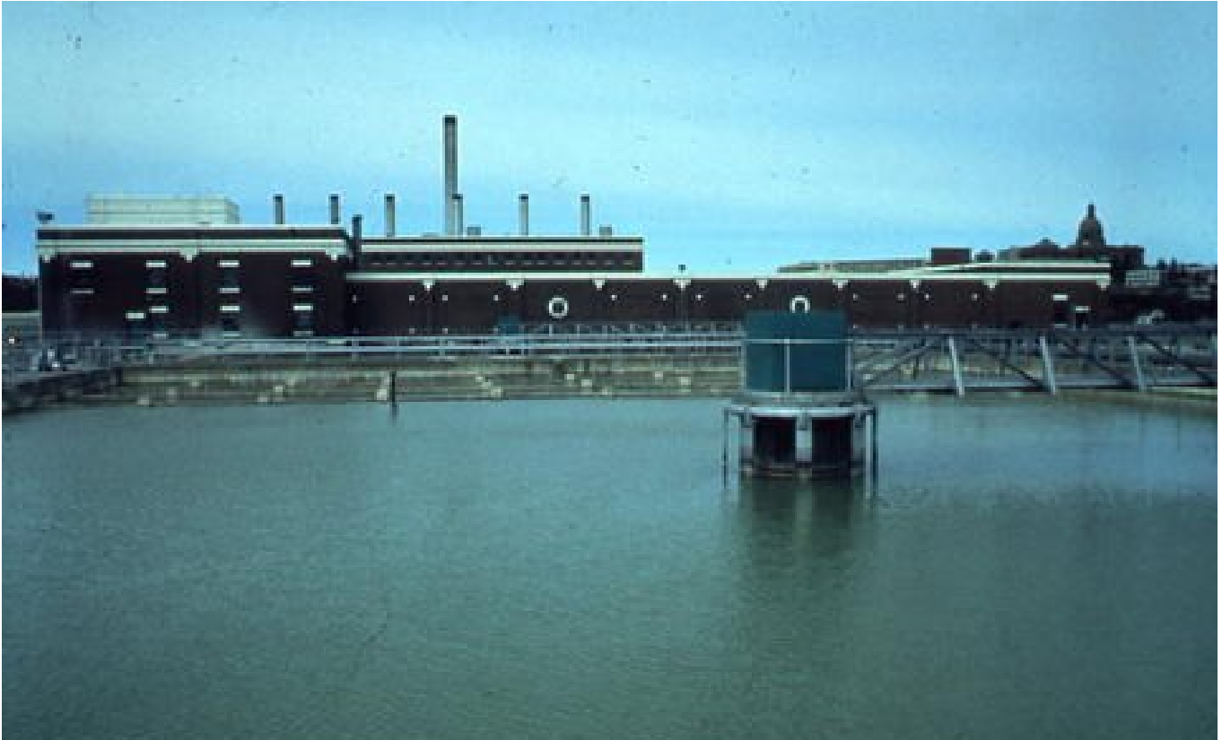
Figure 151: A 1980 view of the water treatment plant in the foreground and LPP behind. (Source: CEA, ET-28-303-141)
