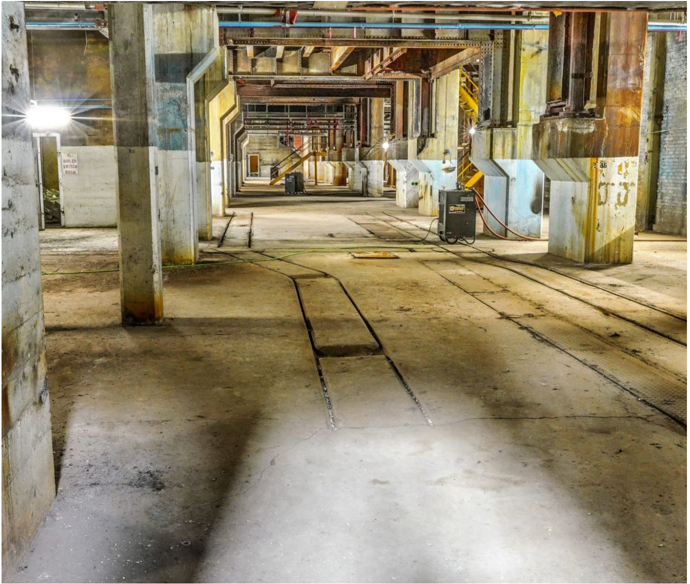
Figure 24: Boiler Hall basement, ash chutes above and ash-car rail tracks below. Note Boiler switch room on the west elevation to viewer's left. (Source: Cloud360, 2020)
