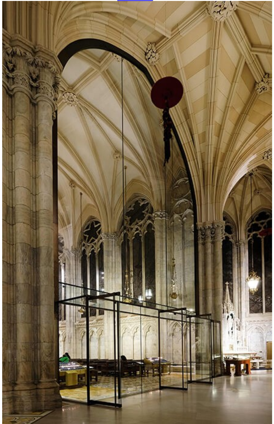
Figure 28: Interior Glass Vestibule for Firebreak/Security/EnergyEfficiency while Maintaining Heritage Views at St.Patrick's Cathedral, NYC (Source: Seele, 2021)
