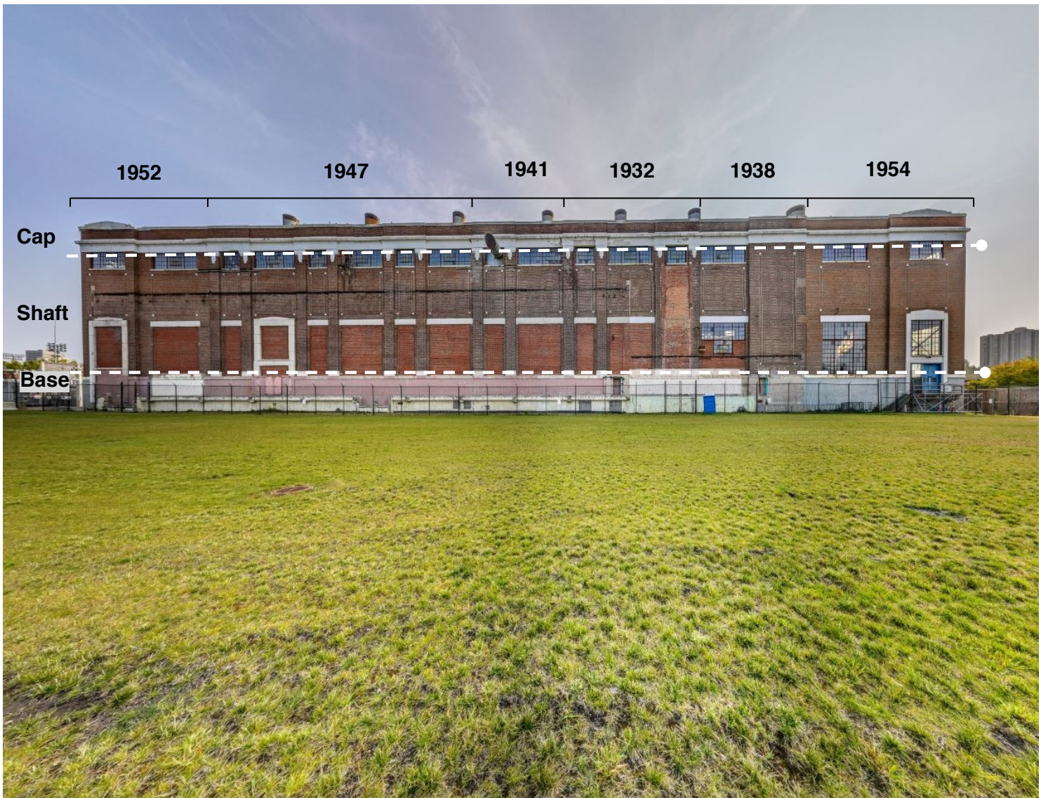
Figure 12: West Elevation of the Boiler Hall with date stamps of incremental additions and windows infilled with brick. (Source: Rossdale Laser Scan Cloud360, 2020)
