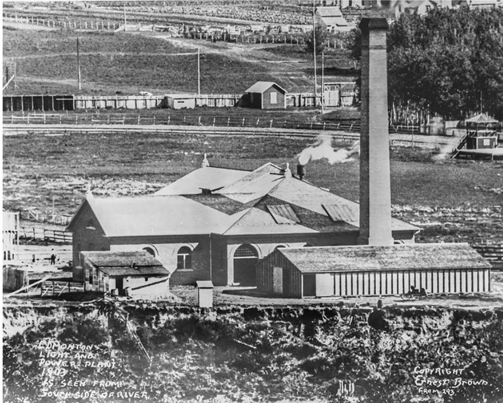
Figure 112: 1903, view of south elevations. (Source: Ernest Brown, EPHF)
