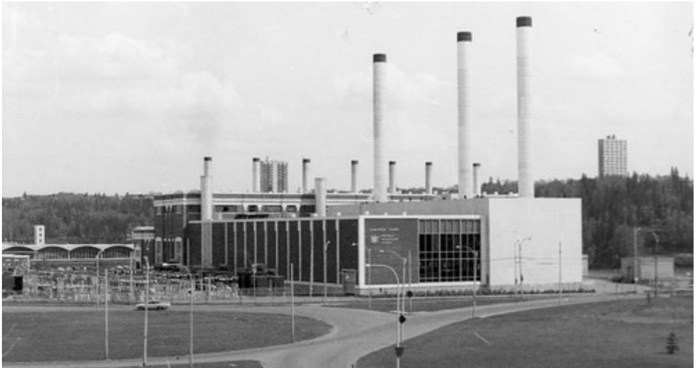
Figure 148: 1976, northwest view of completed high pressure power plant with elevated chimney stacks. (Source: CEA, EA-802-6)
