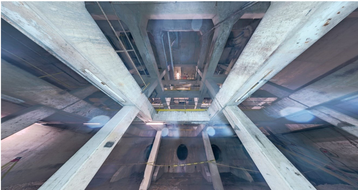
Figure 64: Looking up from the bottom floor of the Dry Well. (Cloud360, 2020)
