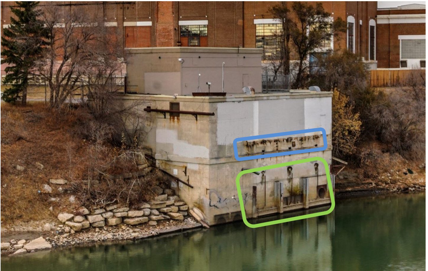
Figure 55: South elevation of Pump House #2 Note evidence of former metal catwalks outlined in blue and partially intact sluice gates and screw jacks outlined in green. (Cloud360, 2020)
