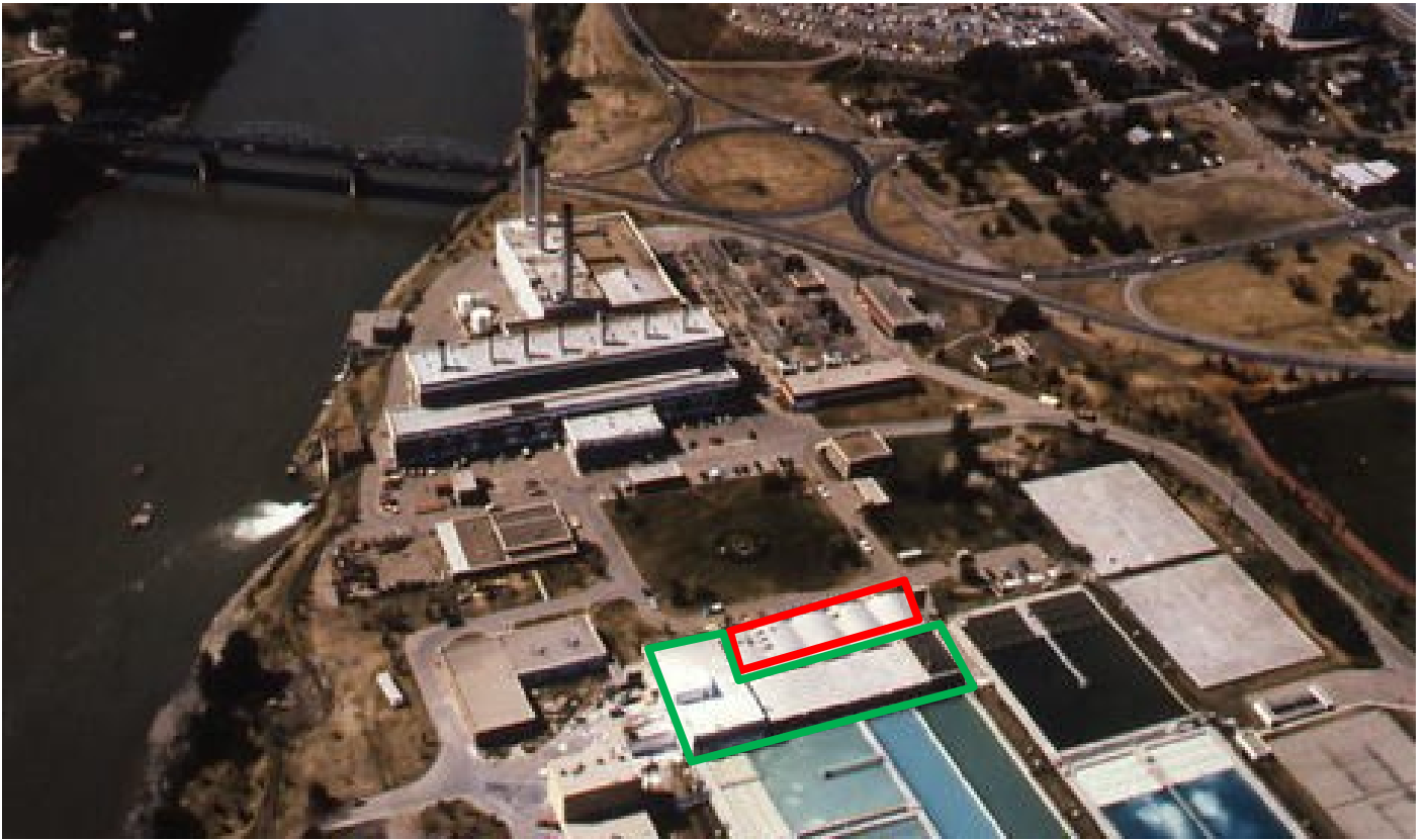
Figure 150: 1980s Aerial view of the site from the west. 1950s addition encircled in red, and the 1940s Dewar design highlighted in green. (Source: CEA, ET-28-302)
