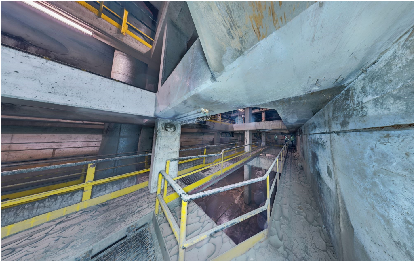
Figure 61: Dry Well Level 3 (Cloud360, 2020)
