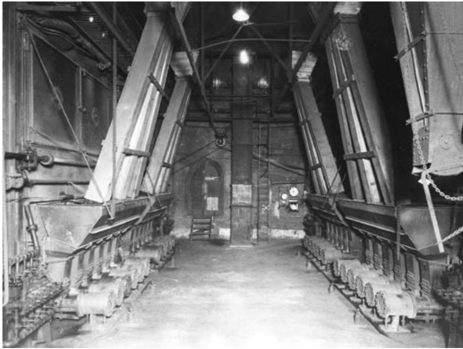
Figure 127: By 1923, up to 16 of the plant's boilers were now fed by hoppers and mechanical stokers rather than by manual hand stoking action. (Source: Glenbow Archives, ND-3-1858)
