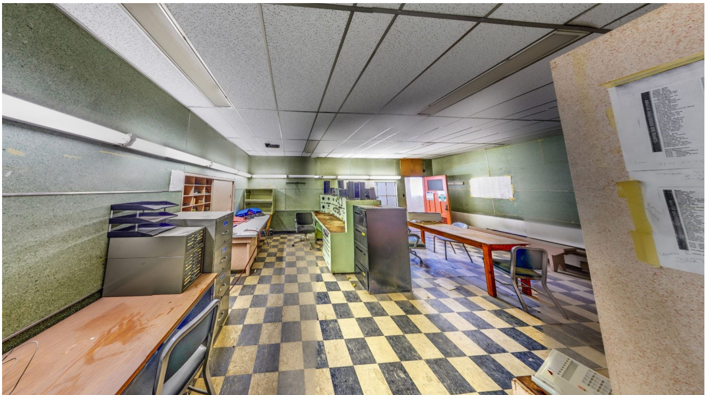
Figure 44: Shift Engineer Office (Cloud360, 2020)
