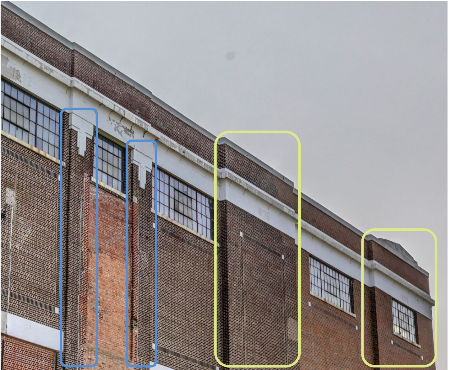
Figure 17: Both the pilasters (highlighted blue) and terminating plant ends (hi-lighted green) extend to 4 brick wythes. (Source: Cloud360, 2020)
