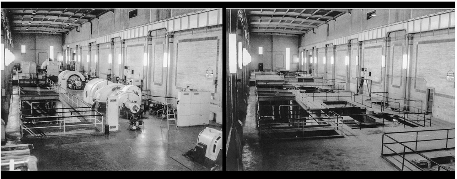
Figure 155: Turbine hall, Units 3, 4, & 5, before and after decommissioning. (Source: EPHF)
