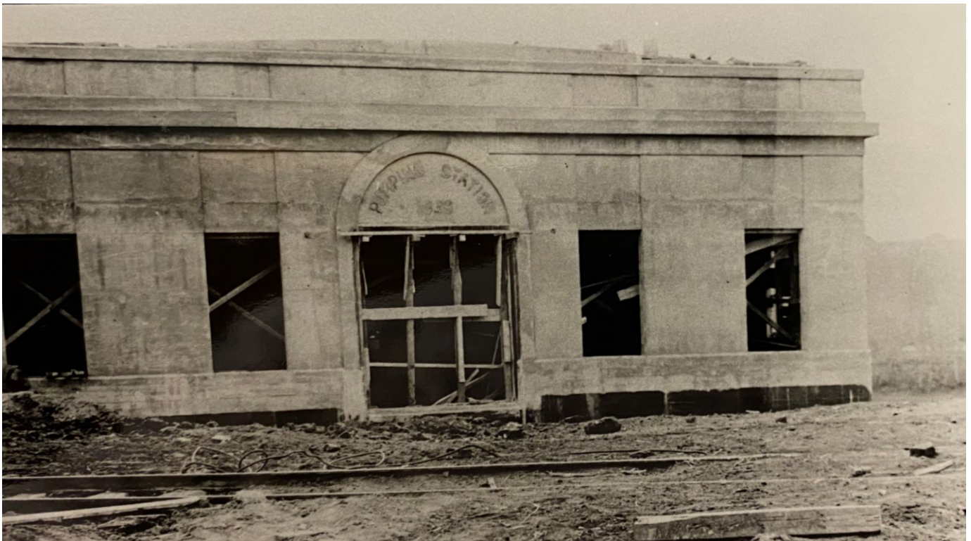
Figure 138: Pump House #1 nearing completion, and before machinery is installed. (Source: CEA, EB-28-1539)
