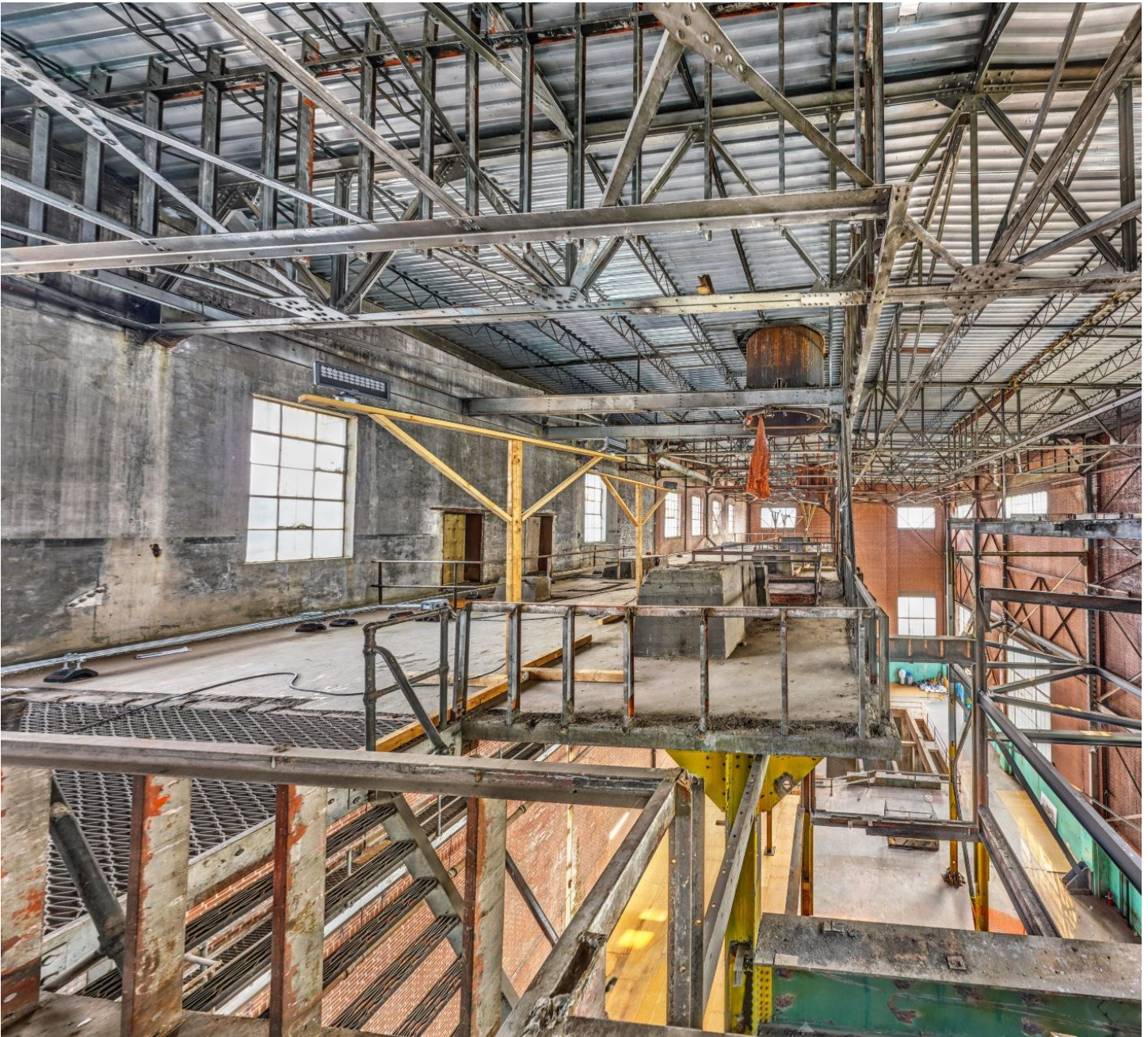
Figure 21: Mezzanine illustrating fan pedestals aligned with corresponding smoke stacks. (Source: Cloud360, 2020)
