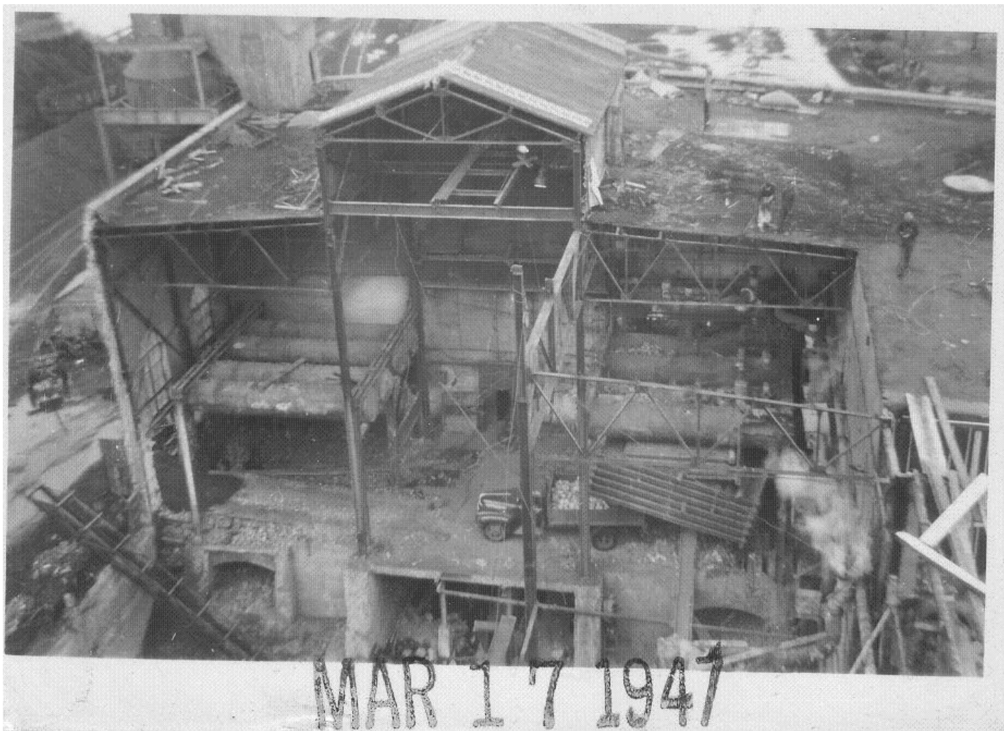
Figure 141: Demolition of part of the last of the earlier power plant, the 1912-13 extension boiler rooms seen here. (Source: EPHF)
