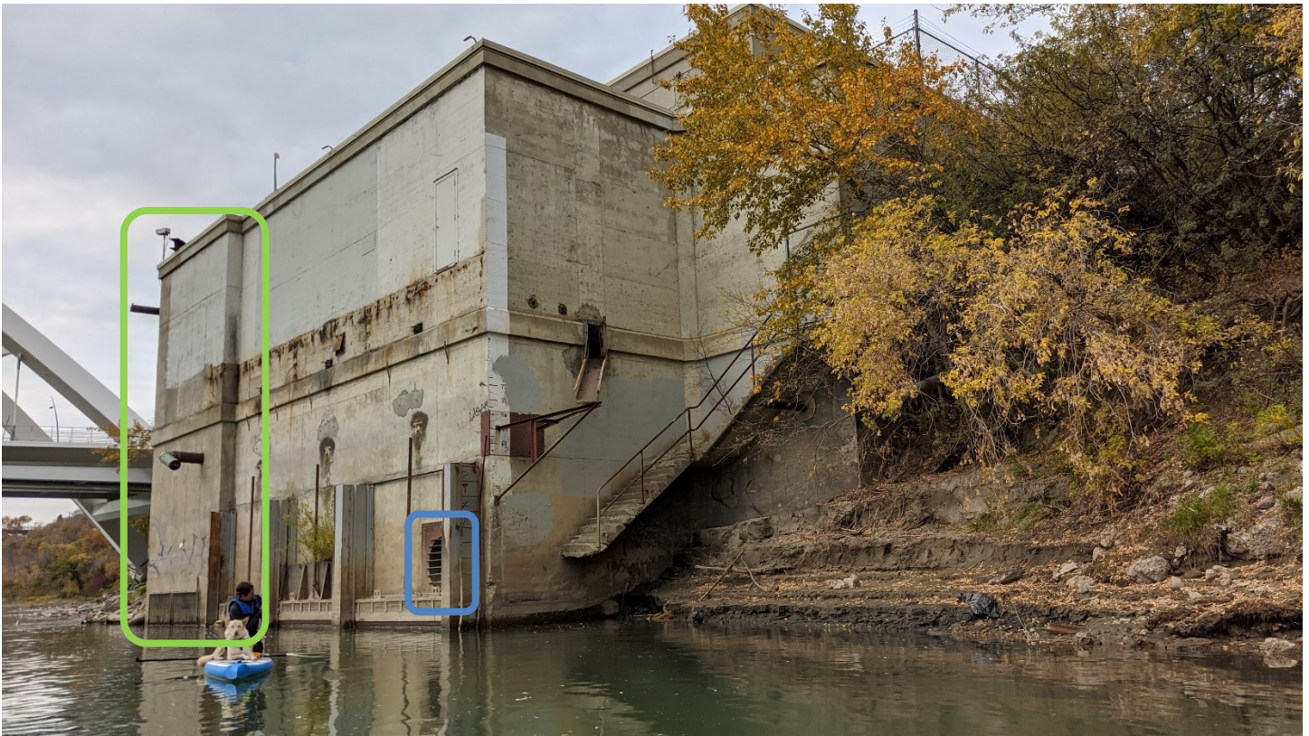
Figure 56: South-east elevation of Pump House #2, note the 1961 wet well addition outlined in green and south-easterly high water intake addition outlined in blue. (Oxland, 2020)
