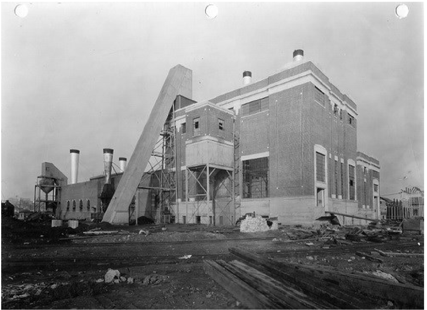
Figure 135: A 1939 south-westerly view of Dewar's Boiler Hall exterior. (Source: CEA, EA-802-1)
