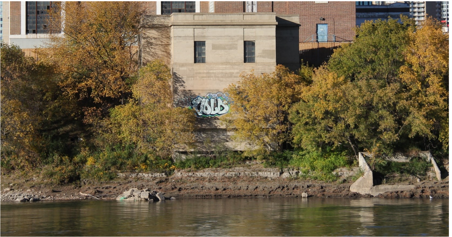
Figure 47: Pump House #1, South Elevation (Source: Oxland, 2020)
