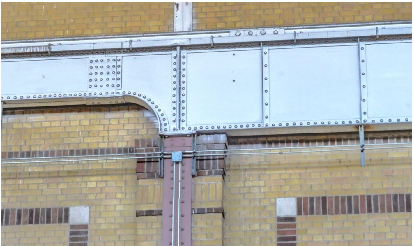
Figure 33: Details of Turbine Hall pilaster capitals, riveted steel, (Cloud360, 2020)
