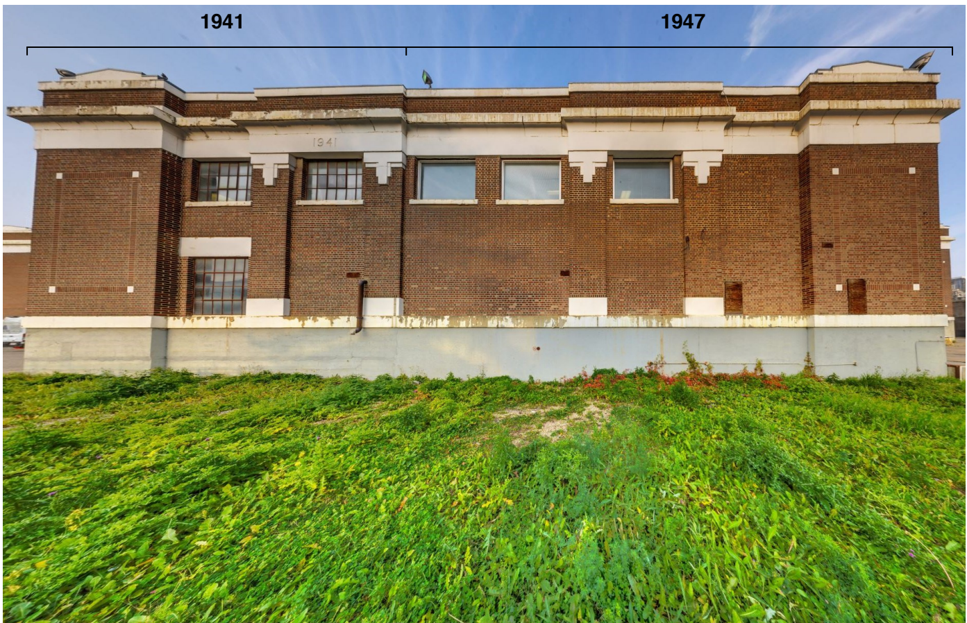
Figure 40: Switch House east elevation (Cloud360, 2020)
