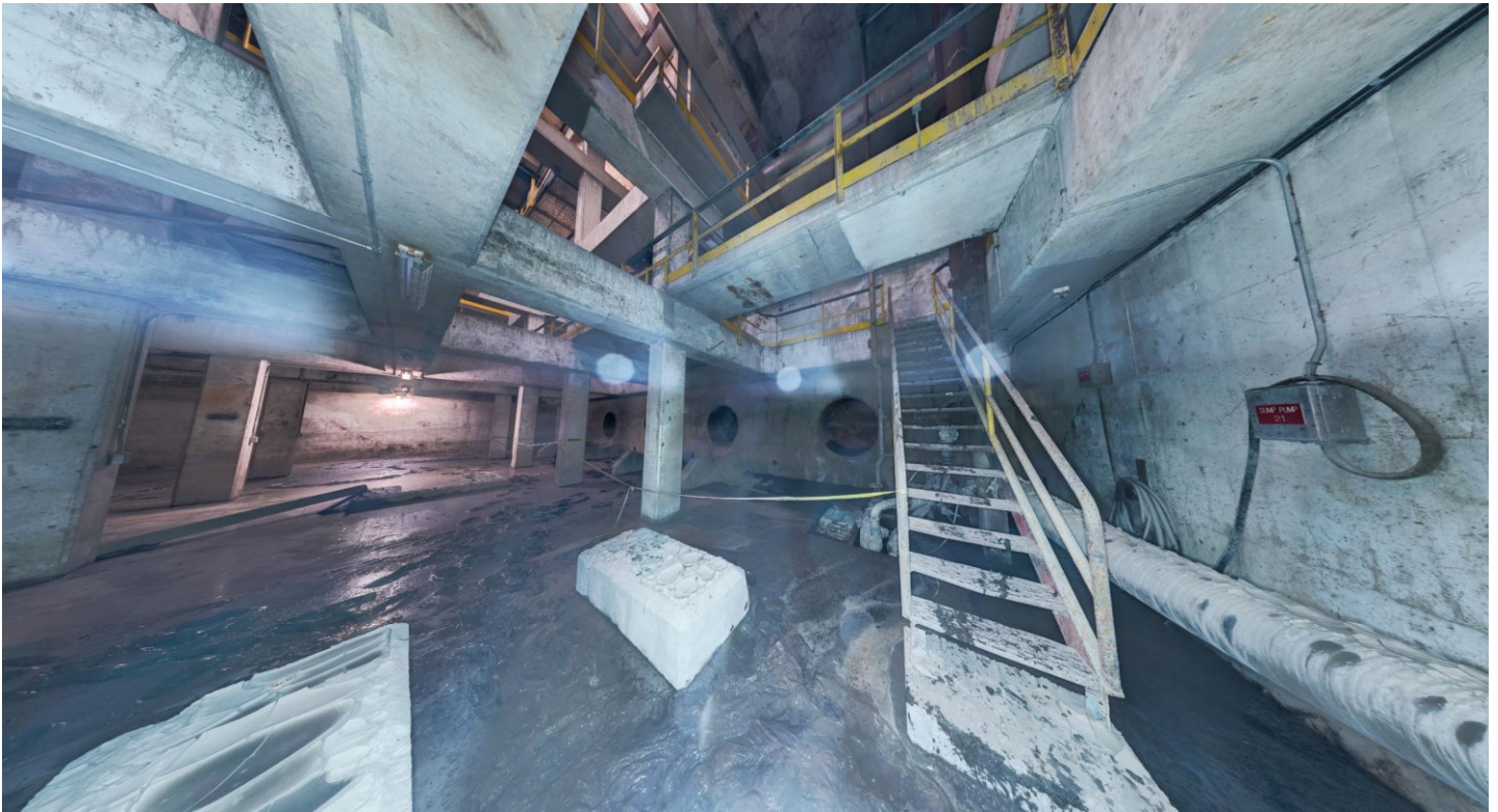
Figure 62: Dry Well Level 4 (Cloud360, 2020)
