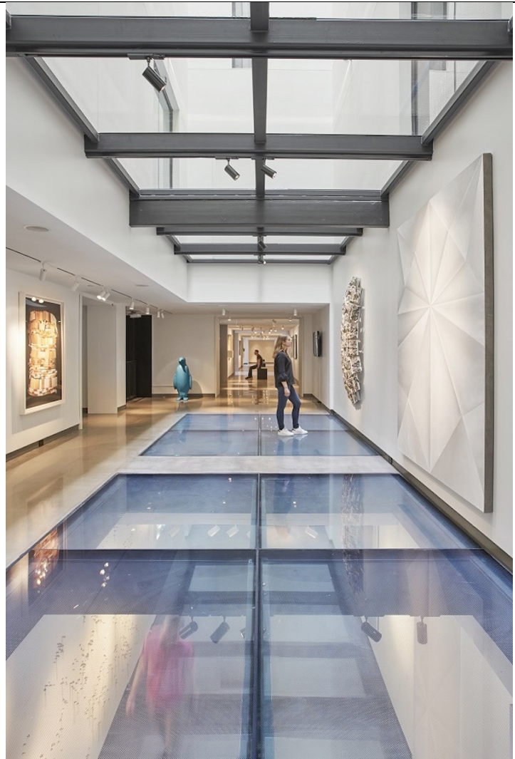
Figure 29: Project 21c Museum Hotel in Nashville, Tenn. features a glass, fire resistive floor. (Source: Building Design Construction Network, 2017).
