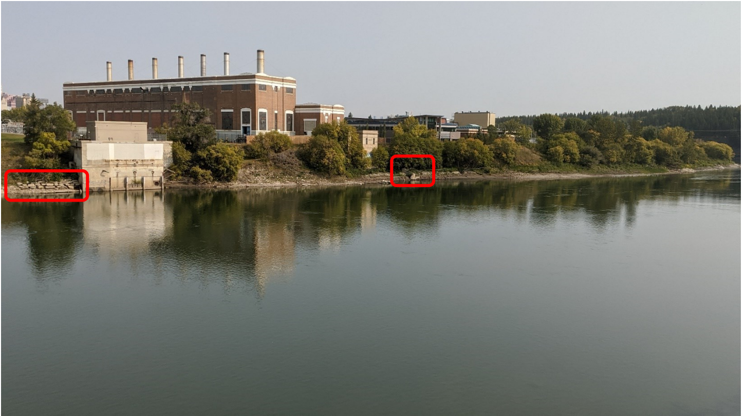
Figure 65: A view of RDPP located along the North Saskatchewan river from the Walterdale Bridge to its south-east. Broken concrete (urbanite) wall and water out-take near Pump House #1 hi-lighted in red. (Oxland, 2020)
