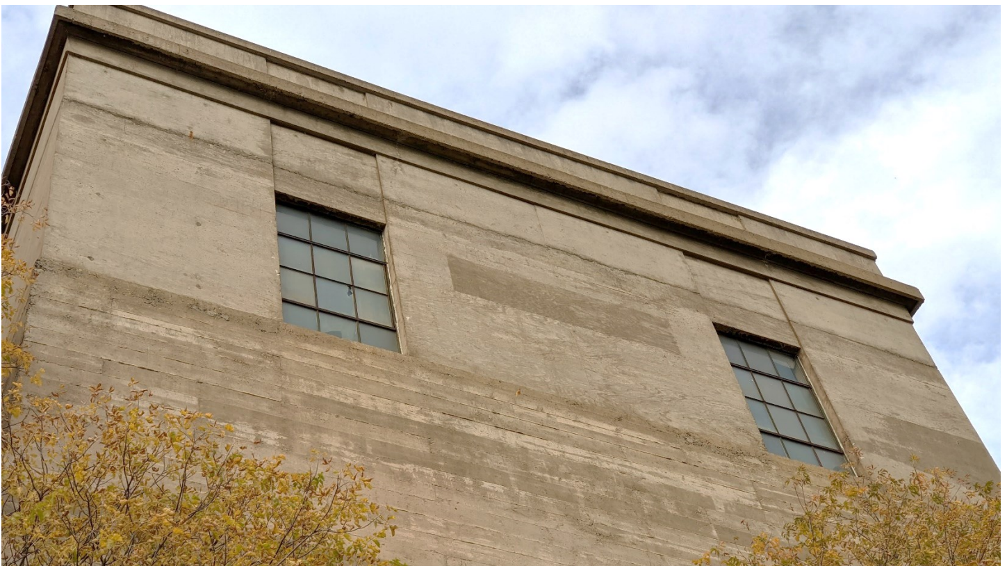
Figure 48: Alternating plywood and board-formed concrete at Pump House #1. (Source: Oxland, 2020)
