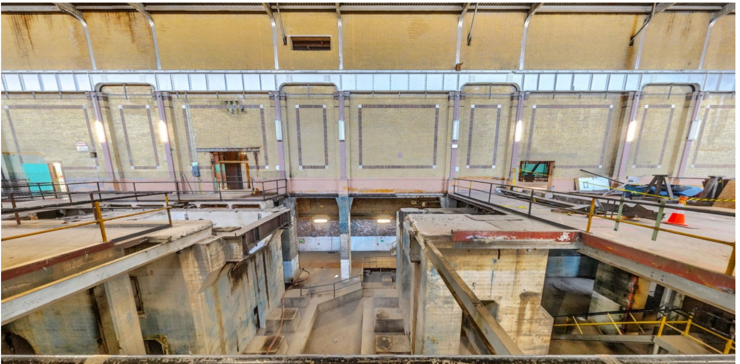
Figure 32: View looking west from the centre of the Turbine Hall of turbine podiums and condenser tank pedestals below. (Cloud360, 2020)
