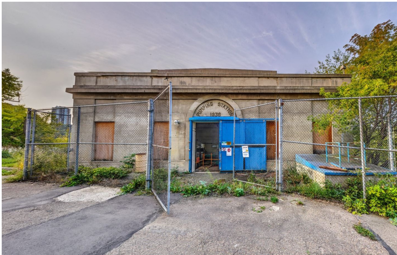
Figure 46: Principal elevation of Pump House #1. (Source: Cloud360, 2020)
