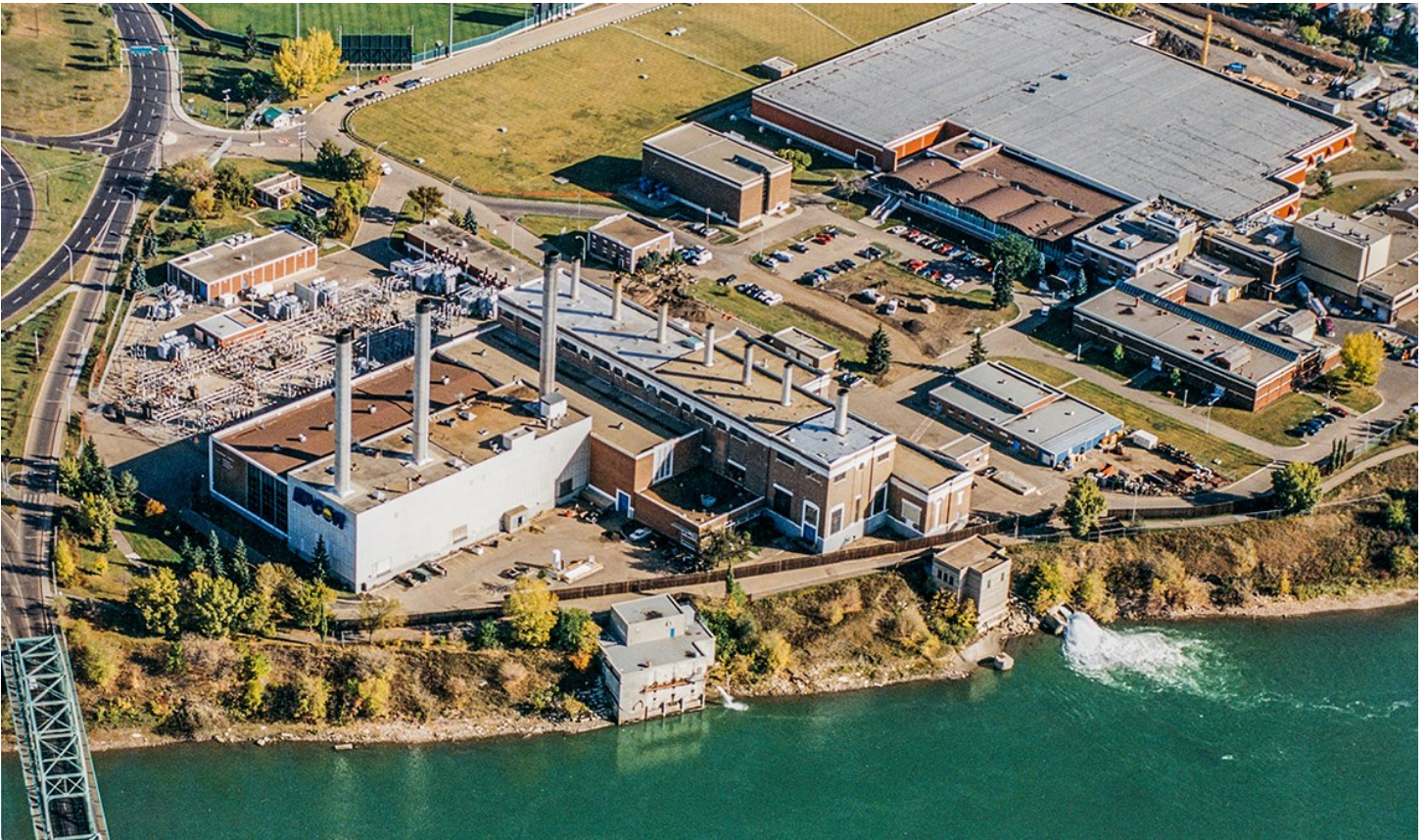
Figure 153: Aerial view of Rosedale Power Plant before HPP decommissioning. (Source: EPHF)
