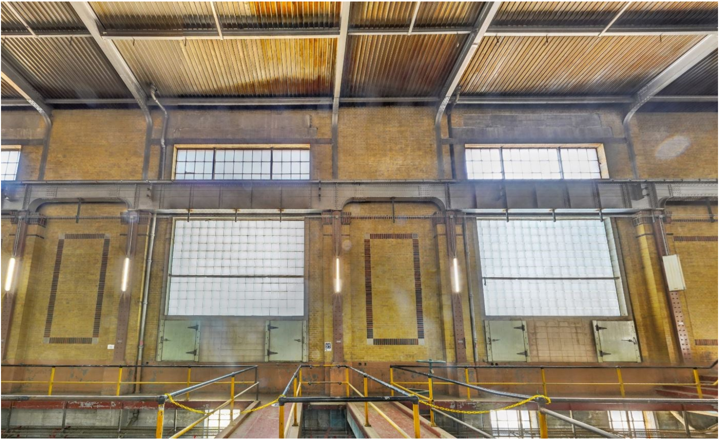
Figure 30: View looking east of lower glass block windows, extant original rolled steel multi-light windows at spandrel locations, and operable louvers at operating floor height. (Source: Cloud360, 2020)
