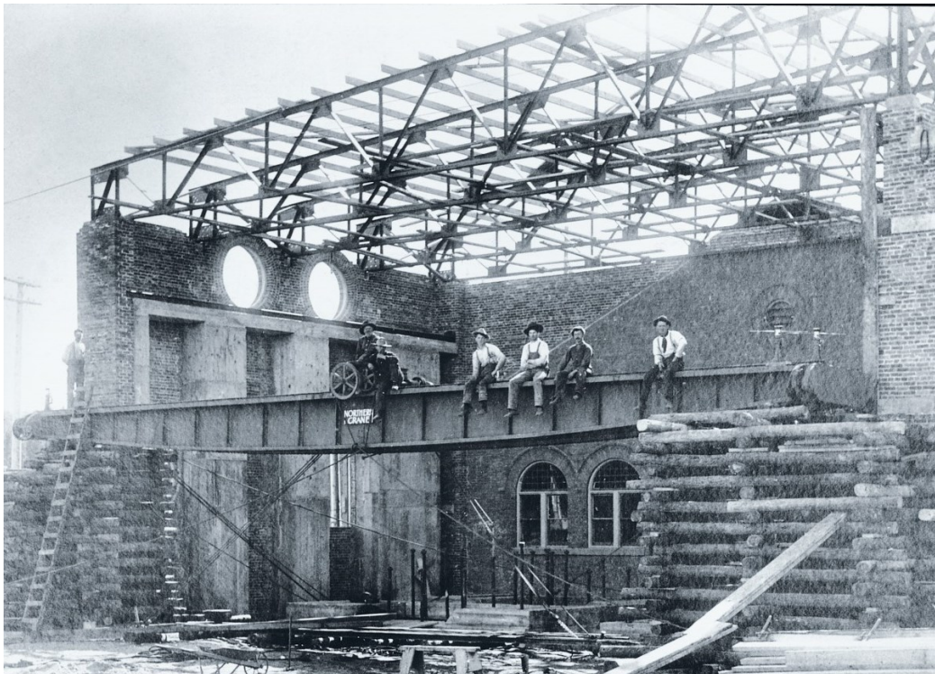
Figure 115: 1906, “Northern Crane” gantry erection using screw jacks and raw timber dunnage in the machinery hall addition on the north end of the 1902 plant. (Source: EPHF)
