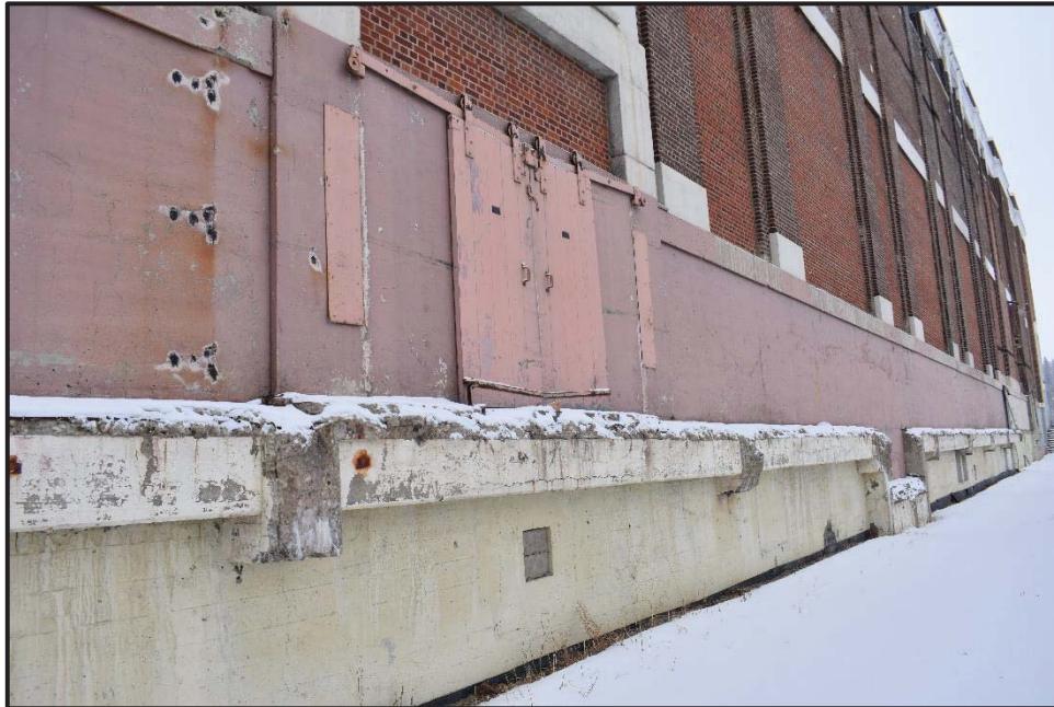
Figure 12-5: Example of Exit Discharge (Exit D8) in Non-Compliant and Unusable Condition
