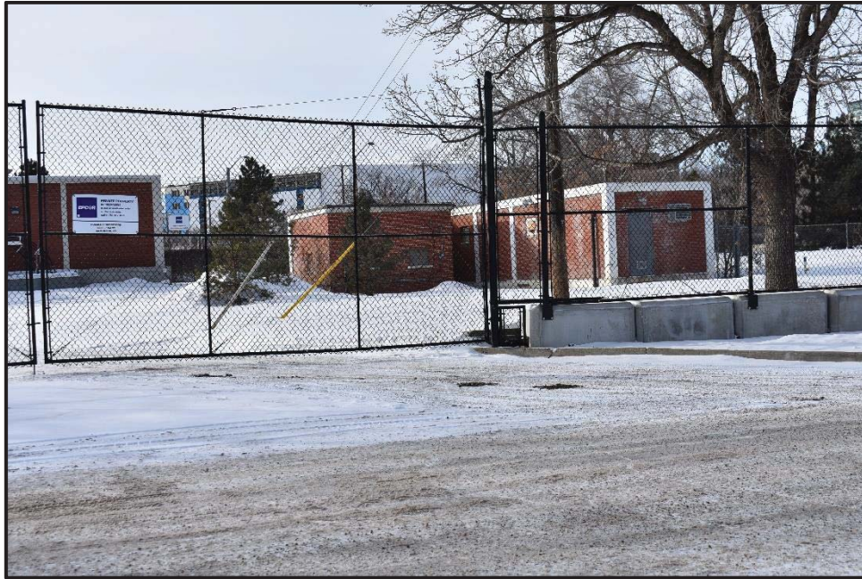
Figure 6-4: ATCO Gas Building Located behind Locked Fencing
