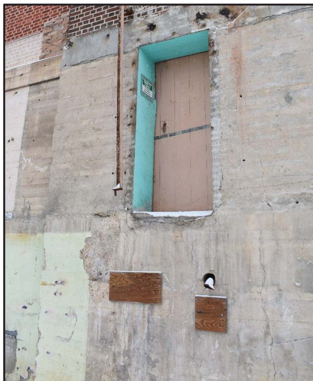
Figure 12-5: Example of Exit Discharge (Exit D8) in Non-Compliant and Unusable Condition
