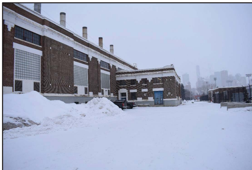
Figure 6-2: Main Site Entrance Requiring Turn-around Facilities
