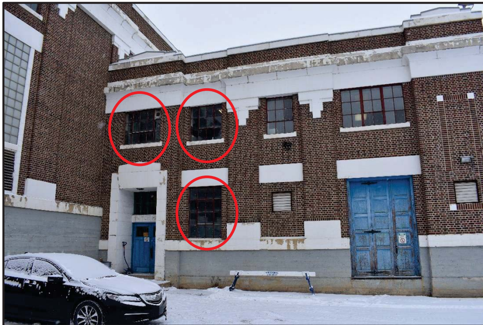
Figure 7-2: Example of Exit Exposure Issues – Switch House (Red Circles)
