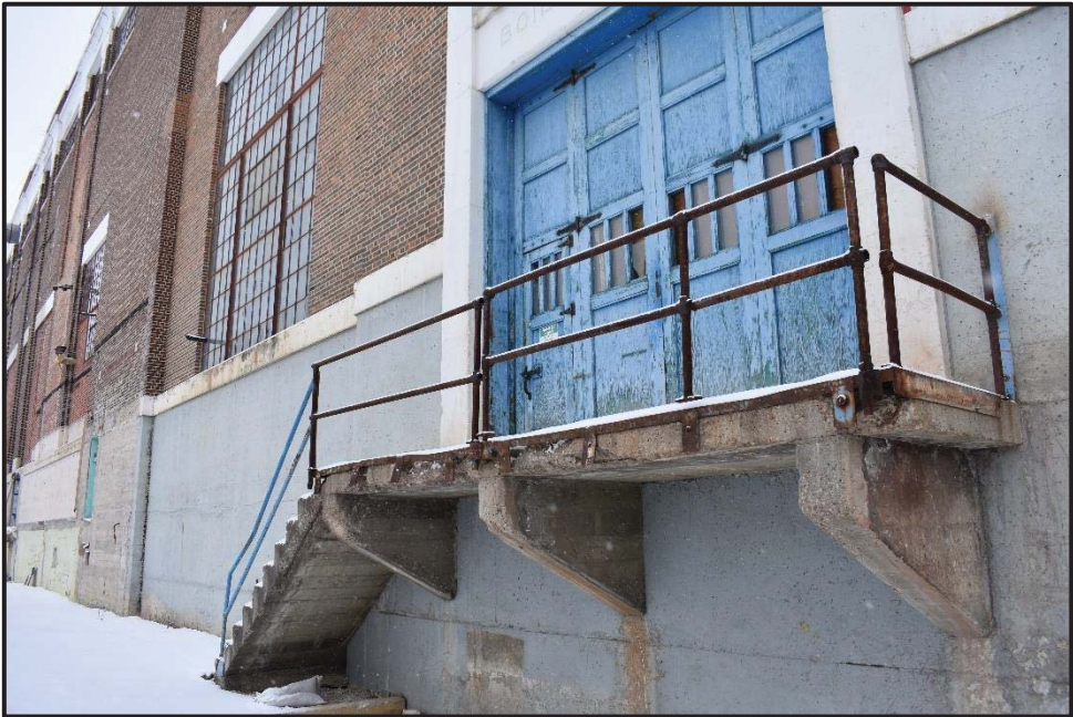
Figure 12-3: Example of Exit Discharge (Exit D9) in Poor Condition and Non-Compliant
