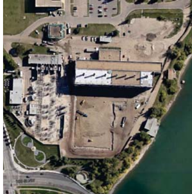
ROSSDALE GENERATING PLANT AERIAL PHOTOGRAPH SCALE: 1:1000
