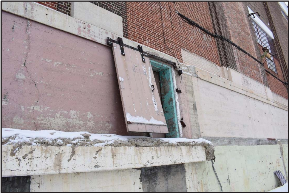
Figure 12-3: Example of Exit Discharge (Exit D9) in Poor Condition and Non-Compliant
