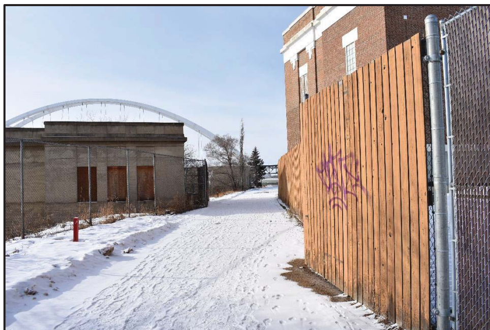
Figure 6-3: Photograph Looking Down Trail Towards Pump House #1 then #2 in the Distance
