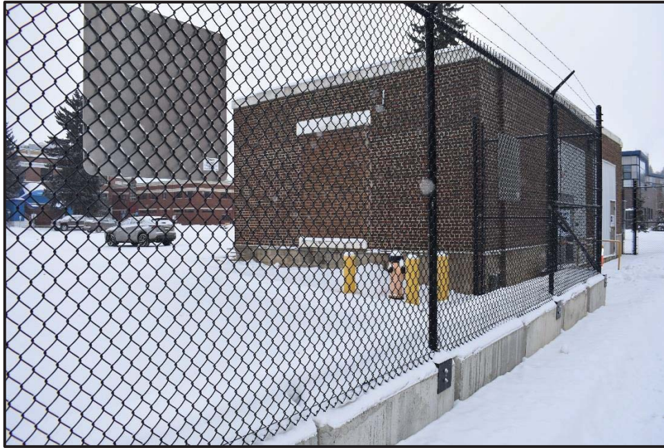
Figure 6-5: Hydrant Location to Project Site Behind Fencing
