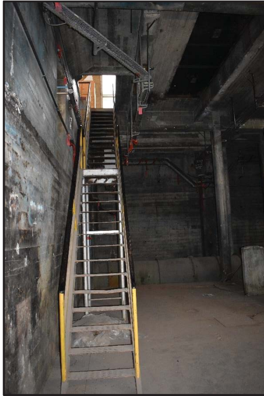
Figure 12-7: Typical Example of Exiting from the Upper Floor Level in Non-Compliant and Unusable Condition
