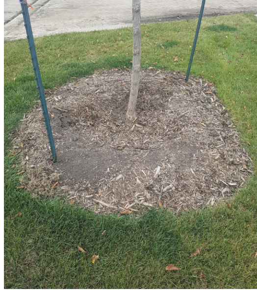
Deficient tree well
