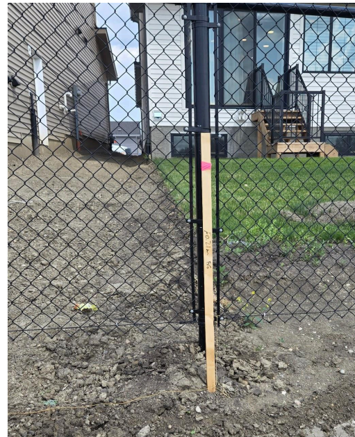
The Inspector may request survey stakes to confirm the intended final grade.
