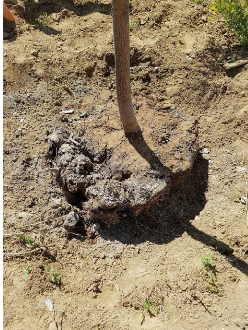
Improper Tree Planting
