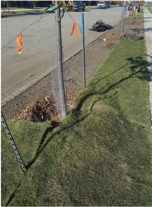
Construction Not Complete
