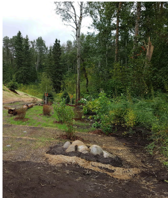
Ready Site (Outfall)
