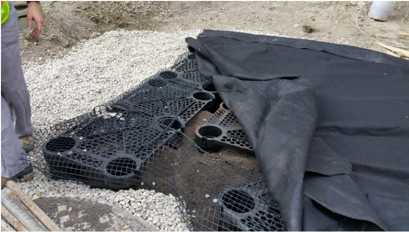
Soil Cell Installation
