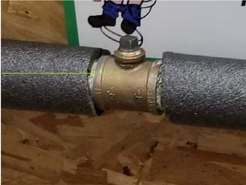
Image 4: Missing insulation
