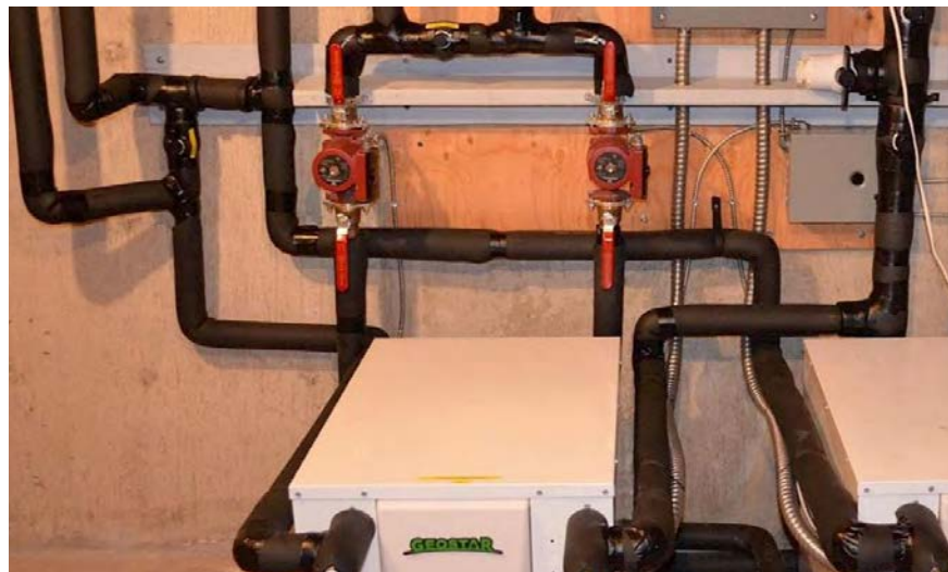
Image 1: Desired Insulation Job
