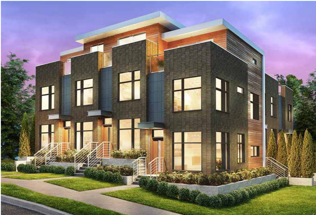
Wood composite provides warmth and colour, and creates contrast with grey brick [24].
