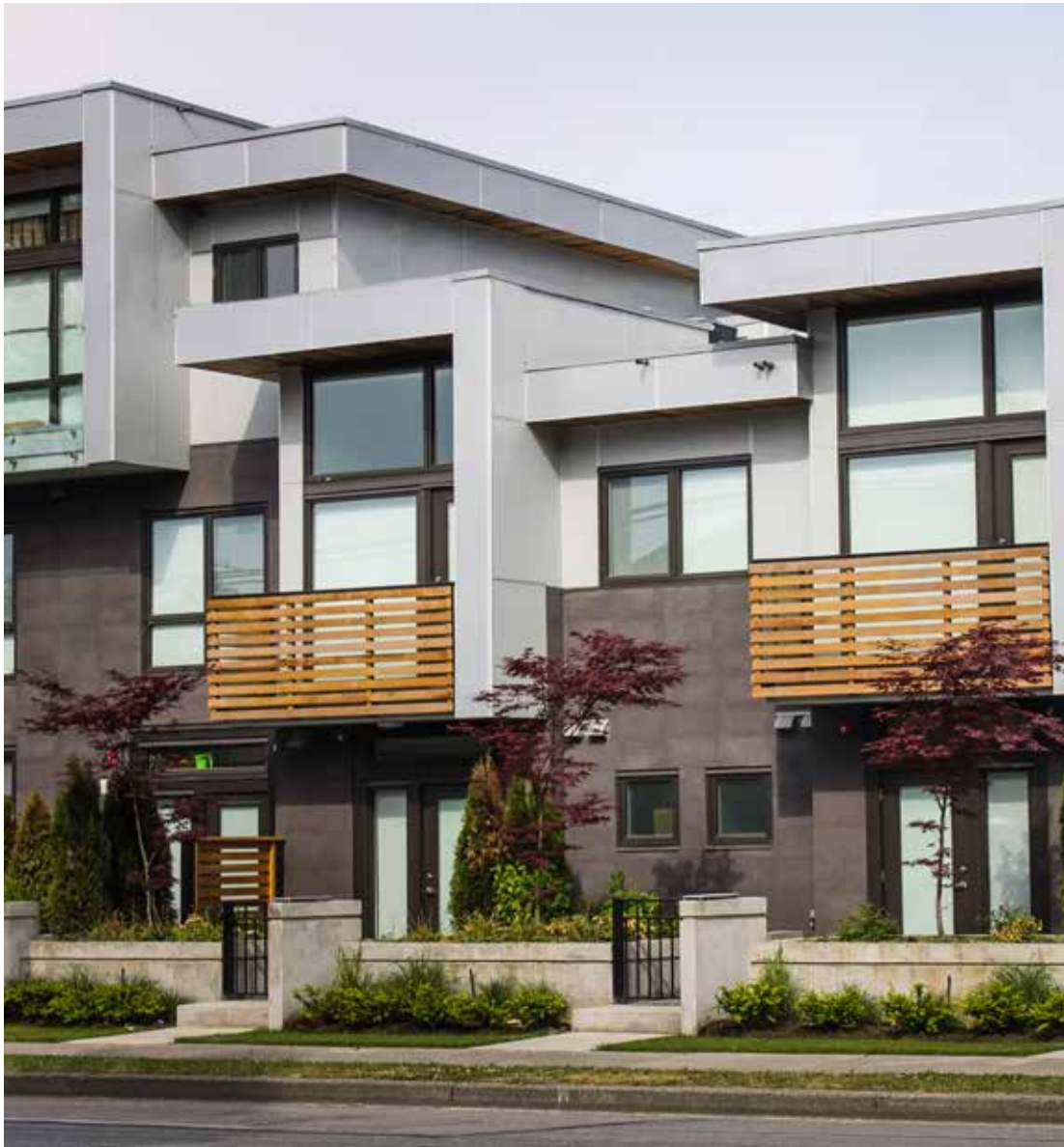
Townhouse design that contributes to the public realm through attractive landscaped spaces within the front setback, street-oriented balconies and a consistent design approach using a limited but compatible palette of materials [2].
