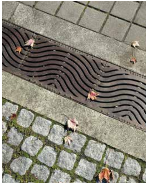
Permeable pavers mixed with other paving material [2].
