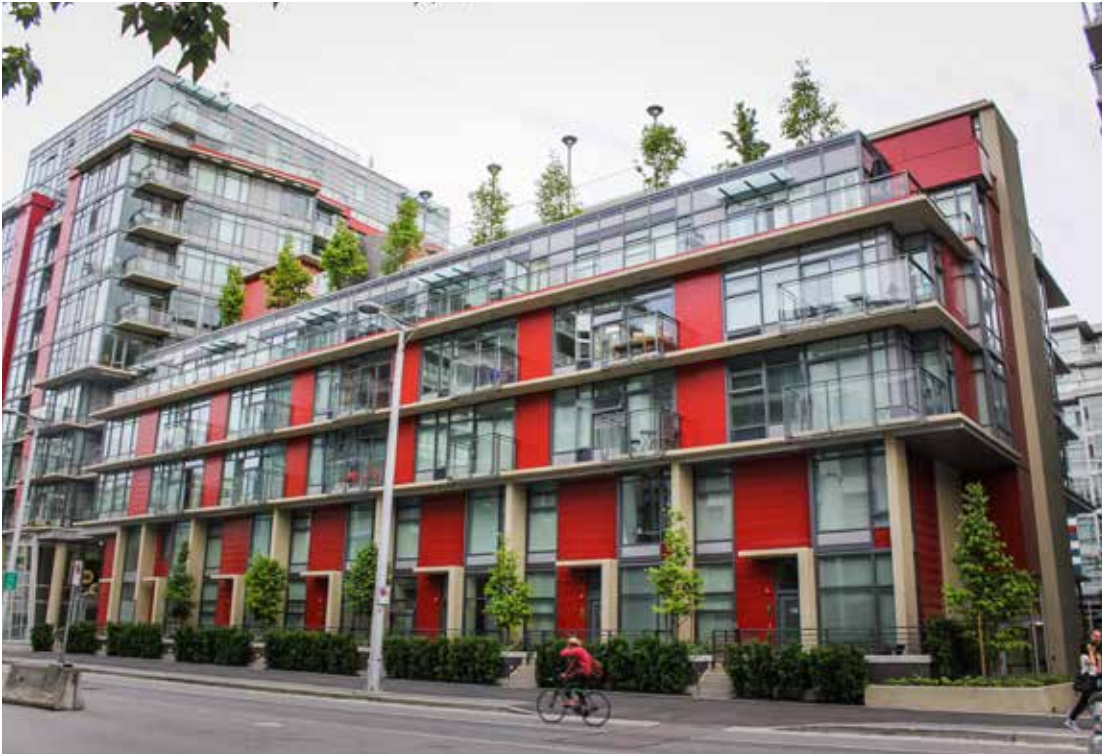
Example of a building with consistent architectural designs on all facade elevations [2].
