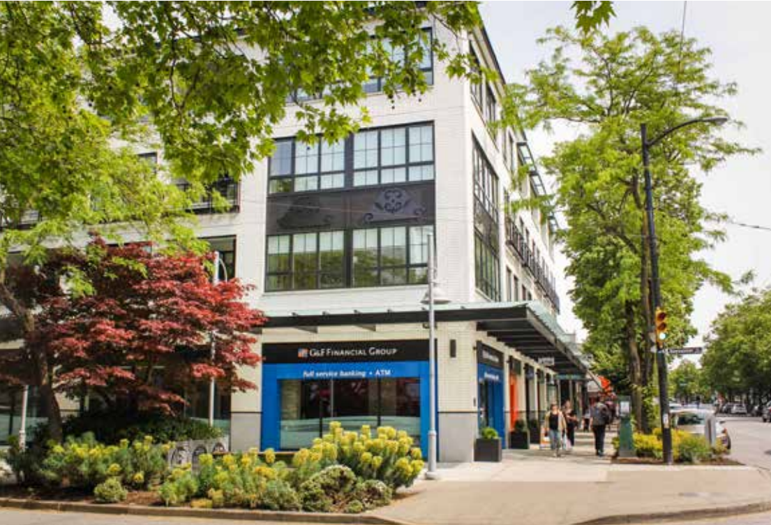
Non-residential frontage expressing individual commercial uses [2].
