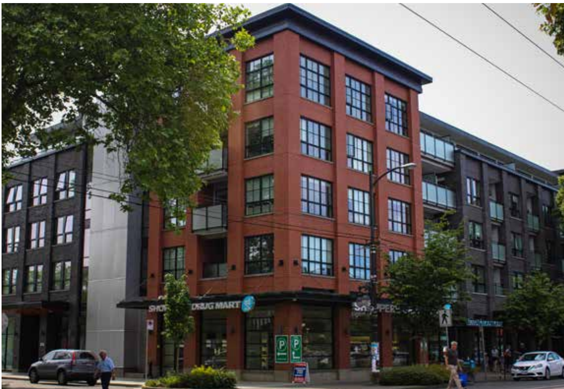
An effective use of demise lines to create transitions in a facade through materials, colour and rhythm, such that a single building has the appearance of multiple buildings, resulting in a more human scale for large buildings [2].
