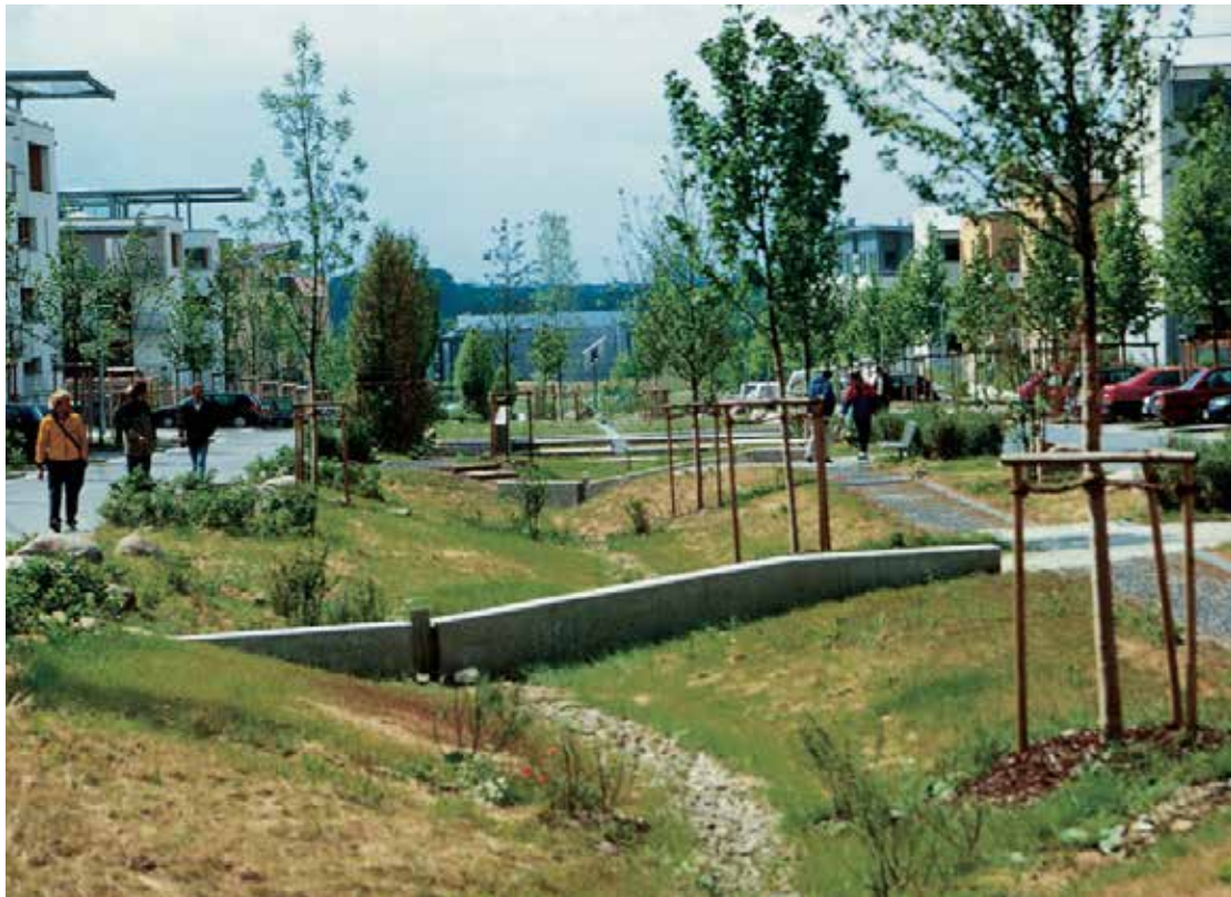
Bioswale to filter and convey stormwater runoff [18].
