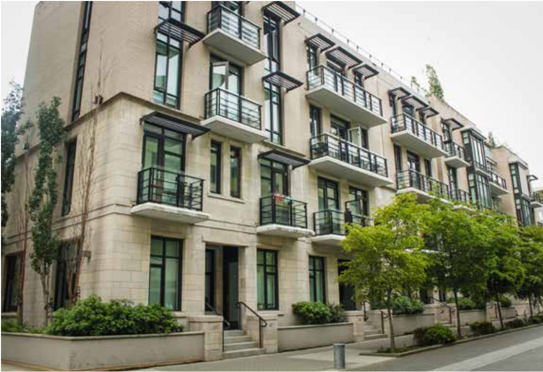
Glazing placement which contributes to the creation of architectural rhythm. Casements and mullions are consistent with other architectural features of the facade [2].
