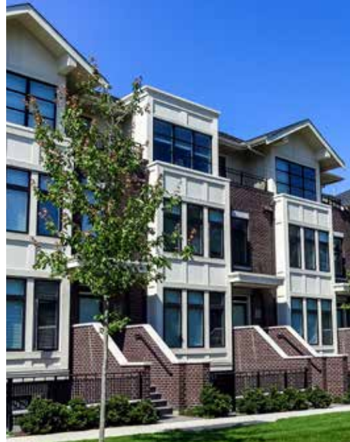
Dwelling fronting a public street with ground floor height separation and buffers to establish privacy [2].
