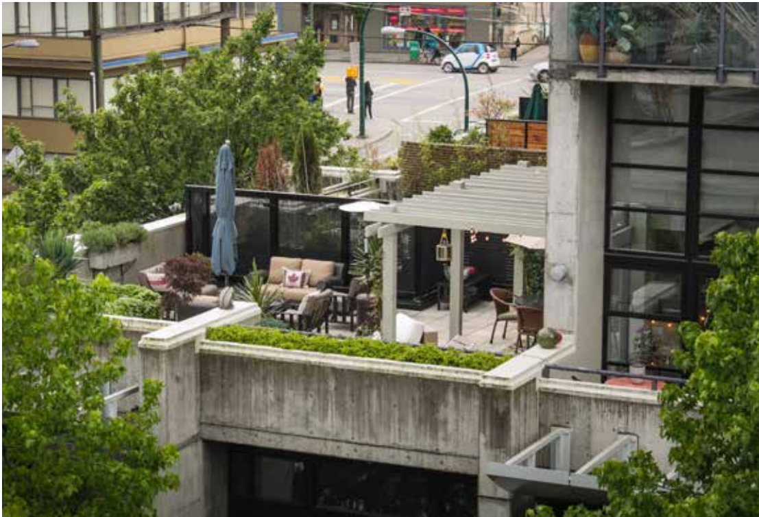
A terrace-level roof amenity space that provides privacy, views and vegetation [2].
