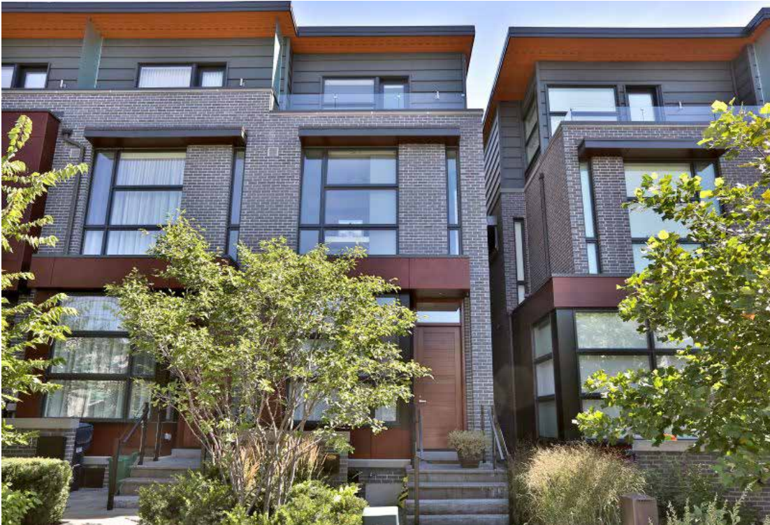
Townhouses that use brick as a primary material, Hardie as a secondary material and architectural metal panels as an accent [23].
