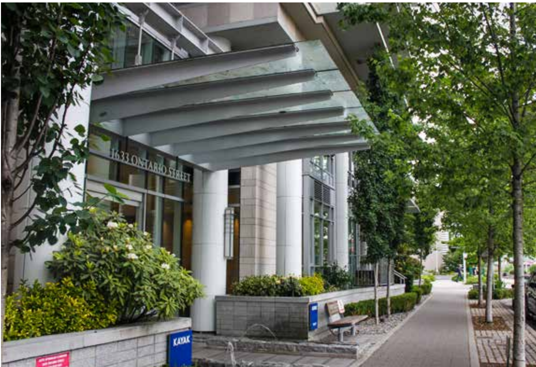
A glass and metal canopy which provides weather protection without blocking sunlight and also clearly identifies the location of the multi-unit lobby entrance [2].
