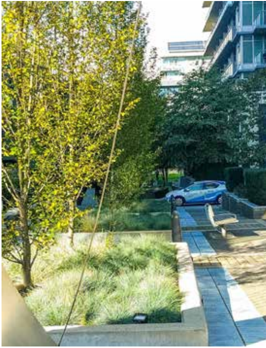
Tree trench box planters support natural irrigation [2].
