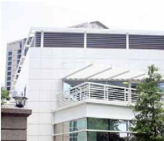
A roof parapet screen that is indistinguishable from the architectural character of the rest of the building [12].
