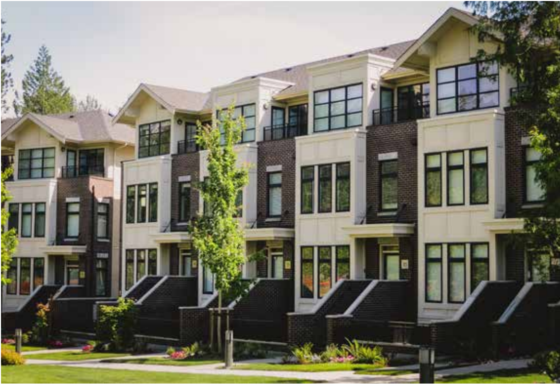
Townhouses with a varied pitched roof design that suits the overall architectural style and provides visual interest [2].
