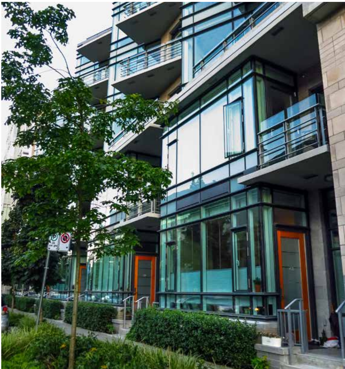
A building oriented toward the street at ground level with a variation in orientation on upper storeys [2].
