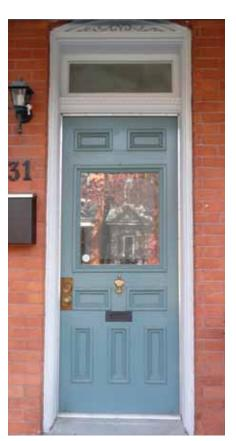
Doors are often targets for replacement because of security, energy efficiency or fire separation needs. Often it is possible to meet all these needs while retaining a historic door. Adding weather stripping can contribute greatly to a door's efficiency. Modern locks and locking mechanisms can often be installed with little damage. The fire rating of a solid wood door may meet certain code requirements.
