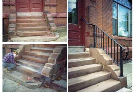
In Rehabilitation, deteriorated features should be repaired, whenever possible, and replaced when the severity of the damage makes it necessary. The stone steps of this house entrance were cracked. Appropriate work included repairing the stone steps and walls and installing a compatible metal handrail to meet building code requirements.
