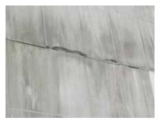
Masonry used on the exterior of modern buildings is generally a cladding attached to a separate structure. Clips, anchors or shelf angles are used to attach the stone panels or brick masonry. The deterioration of these anchors is an area of potential deterioration and failure. Monitoring the condition of these anchors is a vital part of a maintenance plan, as their failure can lead to very significant damage.
