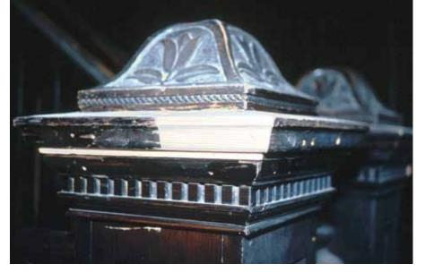
**Wood:** An example of "limited replacement in kind" describes an appropriate scope of work in the Preservation treatment. Only the damaged corner of a stair's newel post at the Commissioner's Residence in Dawson City, has been replaced (it will be stained to match). Only repairing deteriorated parts meant that most of the character-defining elements were retained.
