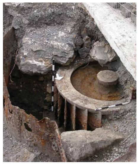
This partially uncovered hydraulic turbine at Pointe-des-Seigneurs, Lachine Canal National Historic Site of Canada in Montreal was installed and used by the Caledonian Iron Works Co. in the late 19<sup>th</sup> century.
