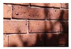
Sandblasting was once a popular method of removing paint from brick; however, it also removed the brick's outer hardened "crust" causing the brick to deteriorate.
