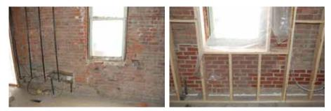
Left: Interior of west (rear) wall of north retail bay, showing as-found condition of load-bearing masonry after removal of the lath and plaster interior finishes for inspection purposes. Uncontrolled runoff from the roof had saturated the wall, washed out the mortar, and caused localized collapse around the window opening.
