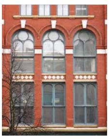
These large windows on King Street in St.John were originally slated for removal and replacement as part of the CentreBeam Place rehabilitation project. Instead, a condition revealed that the original windows could be retained and repaired, with the addition of interior storm to meet energy efficiency requirements.
