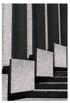
Special formwork or chemical or mechanical treatments can create a wide variety of concrete finishes, such as these pre-cast panels with exposed Laurentian granite aggregate at the National Arts Centre in Ottawa. Recreating these finishes when repairing or replacing-in-kind should be preceded by a mock up to ensure that the new work will be compatible with the historic place.
