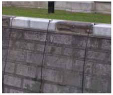
Masonry: In this rehabilitation project of the Rideau Canal, some of the original limestone blocks remained in good condition. Others, which were too deteriorated to repair, were replaced in kind with new limestone blocks.
