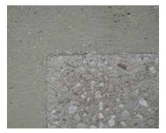
Important properties to match when patching concrete can include the modulus of elasticity, cement to aggregate ratio, aggregate gradation, compressive and shear strength, and coefficient of thermal expansion. In this case the coarse aggregate in the repair patch does not match that of the original concrete.
