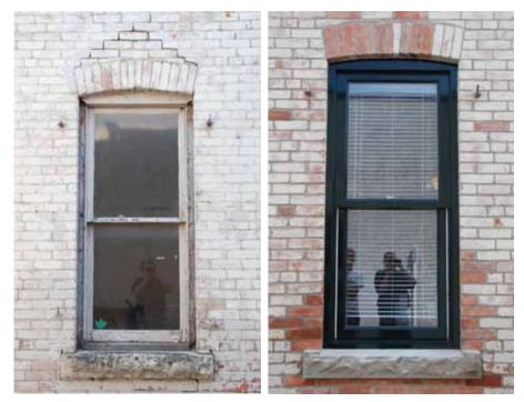
Left: North façade window prior to rehabilitation showing eroded mortar joints, cracking due to frost action within the wet wall, and delamination of the sandstone sill.
