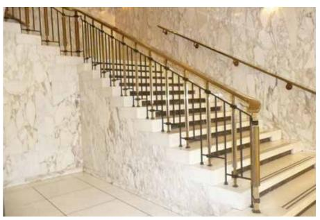
Historic guards and handrails often do not conform to current codes and safety regulations. Modifying historic balustrades in a compatible way to meet these requirements is recommended over replacement. The balustrade at the National Archives and Library in Ottawa underwent a sensitive rehabilitation to meet current requirements for spacing between balusters.
