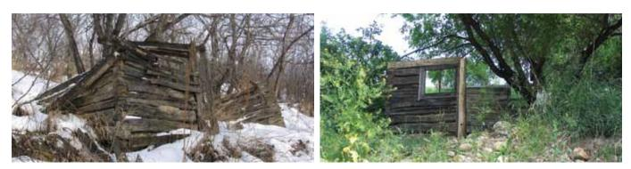
The character-defining elements of Doukhobor Dugout House NHSC in Saskatchewan, such as the window frames, had suffered visible deterioration from exposure to the elements. A long-term repair solution was necessary to prevent further decay and to preserve the site's heritage value.
