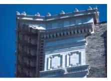
One of the primary causes of deterioration of glazed architectural terra cotta, like that shown on the Confederation Life Building in Winnipeg is water. Water-related damage to the glazed units, mortar, metal anchors or masonry backfill can be repaired only after eliminating the sources of that water. In order to ensure that the actual root problem is being solved, investigation work would need to be completed prior to any repairs in order to identify that source.
