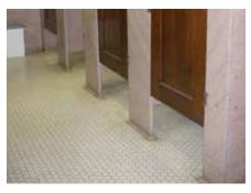
Mass-produced elements, such as ceramic tiles, are frequently used in buildings. Finding matching replacements for repair work can be almost impossible. If tile needs to be removed from one area, it is good conservation practice to save nd stockpile it for later use elsewhere in the building. These tiles from the washrooms in Union Station in Toronto were removed from one set of washrooms in order to provide a stockpile of tiles to use in the repair of the remainder of the washrooms.
