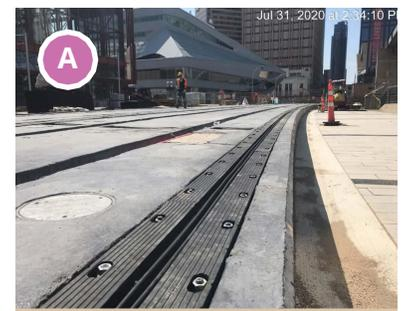
*Floating track slab rail installation (TransEd)*
