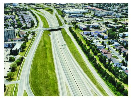
Even using a service road concept, there is insufficient space to develop both on-and off-ramps at all interchange locations.
