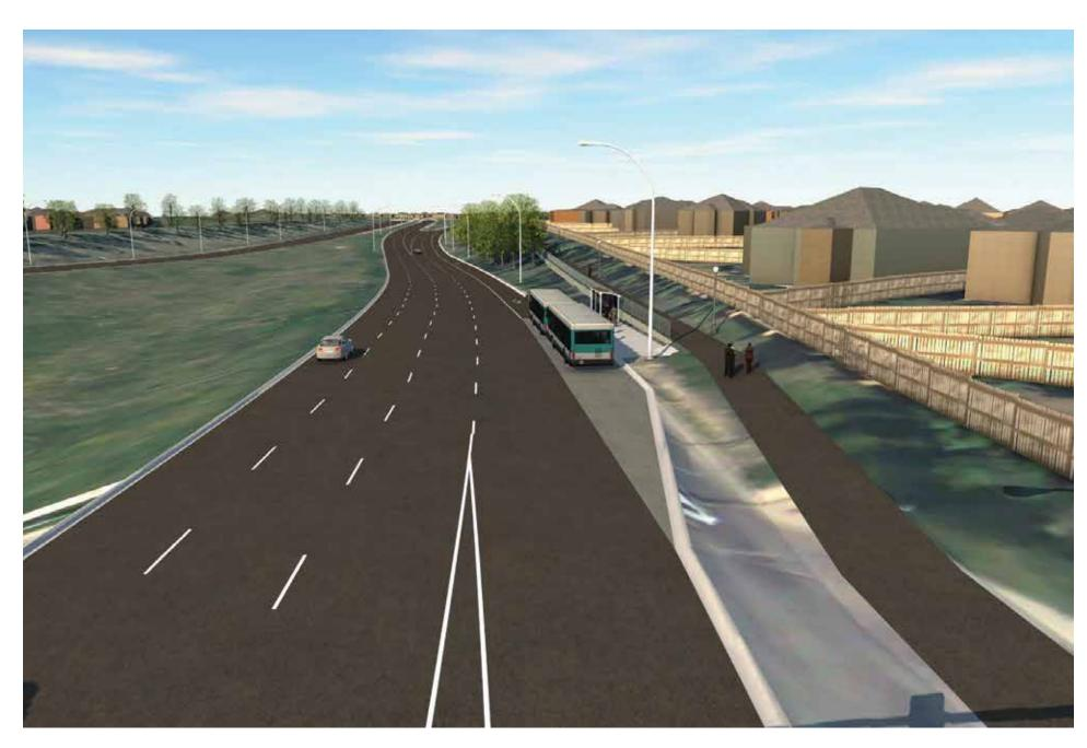
Concept of the separated bus lane at a bus stop.
