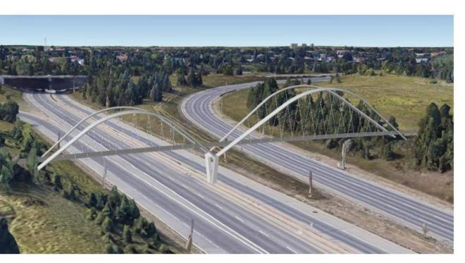
Thin deck hung from steel arch with one pier
