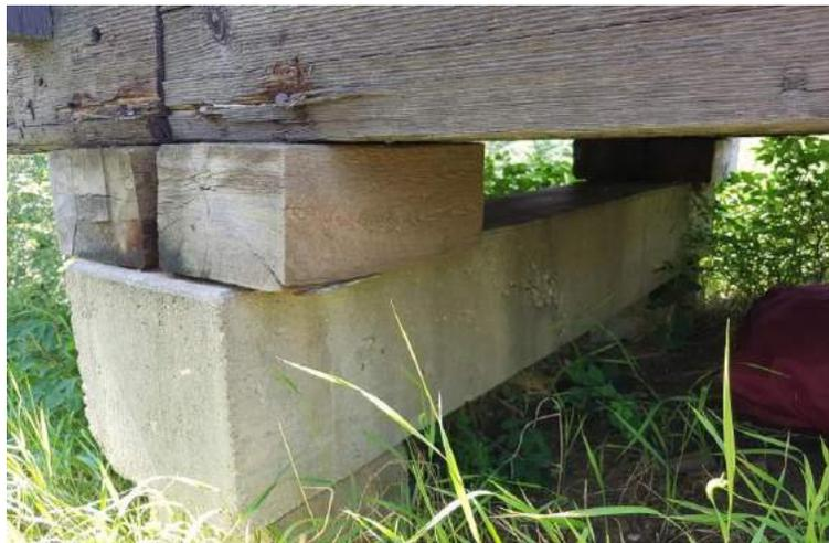
**Plate 8. End of first span and associated foundation near northern terminus of existing pedestrian trestle bridge.**
