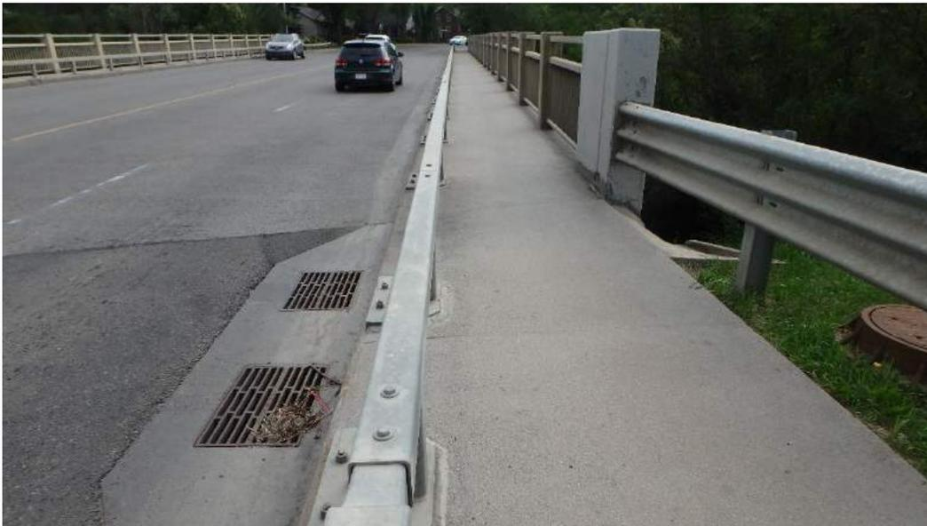
**Plate 3. View east showing drainage CBs adjacent to southwest sidewalk on SPR.**
