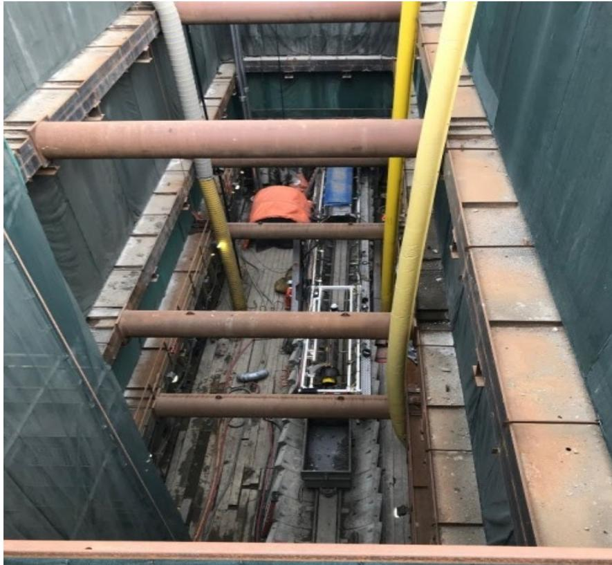
**Figure 2d – SESS SA10a, Working Pit and Installation of Tunnel Boring Machine**
