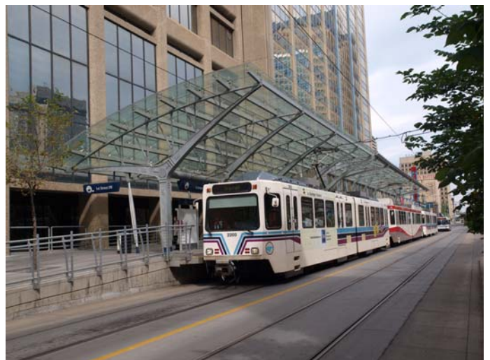
A high-floor LRT station integrated into a building in downtown Calgary, Alberta
