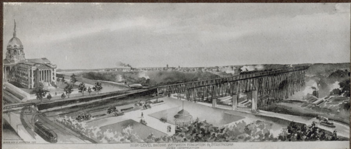
HIGH-LEVEL BRIDGE BETWEEN EDMONTON & STRATHCONA UNDER CONSTRUCTION
