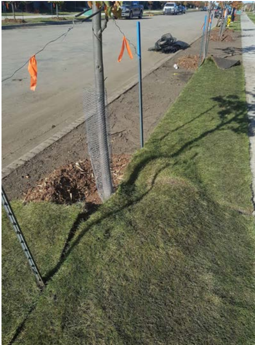
Construction Not Complete
