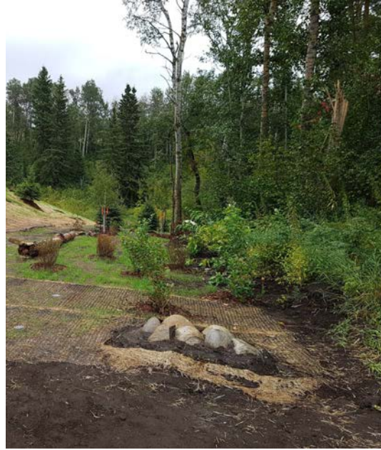
Ready Site (Outfall)
