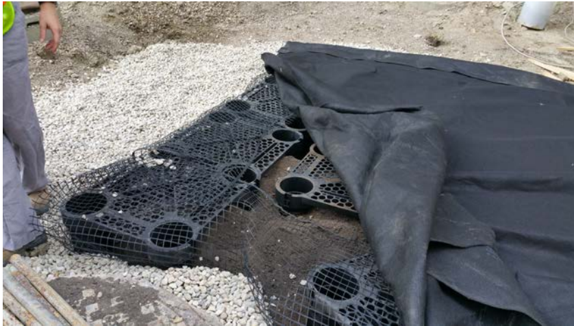
Soil Cell Installation
