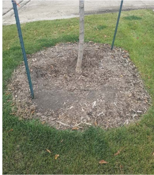
Deficient tree well
