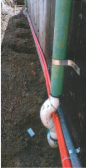
**Figure 6 |** Rainwater leads must go around the electrical conduit
