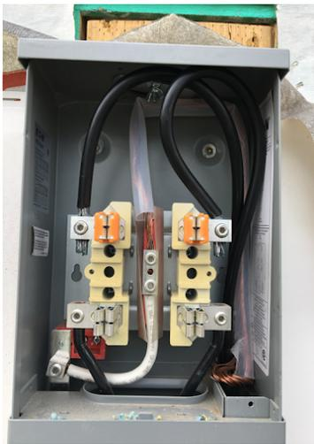
**Figure 9 | Alternative Meter Base Configuration**
