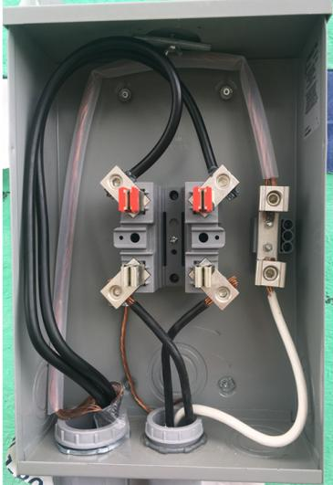
**Figure 8 | Alternative Meter Base Configuration**
