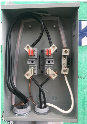
**Figure 10 | Alternative Meter Base Configuration**
