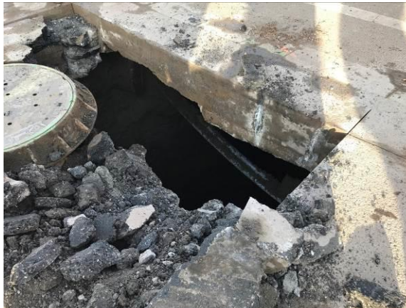
Figure 2.0-2 Severe Deterioration of 61 Avenue Trunk
