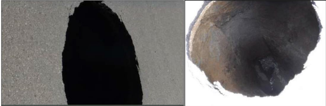
Figure 2.0-6 Pictures of Sinkhole at Lauderdale
