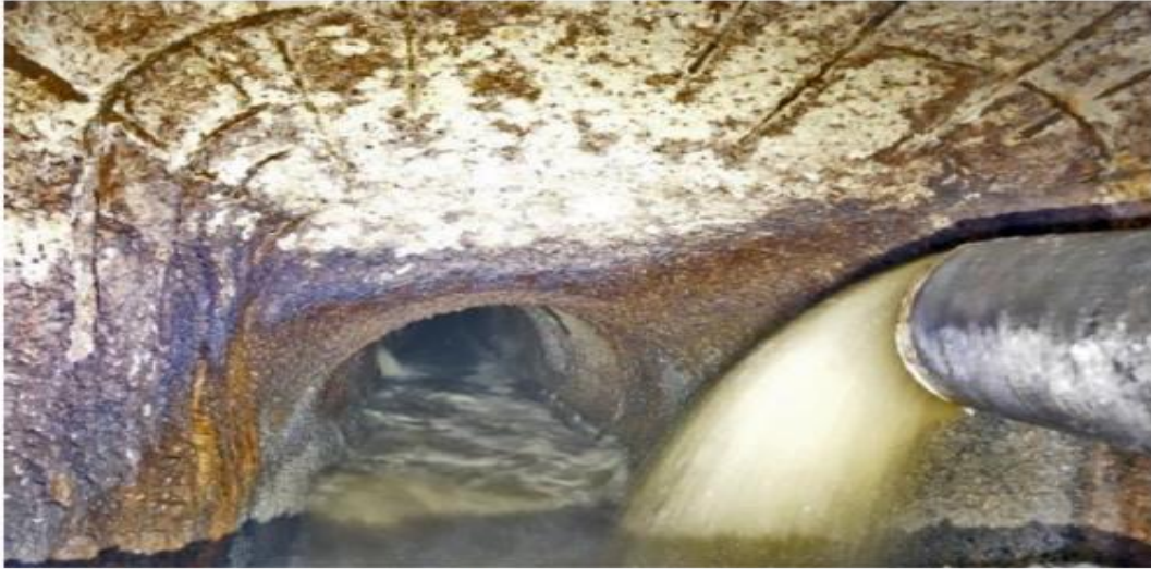
Figure 2.0-5 Duggan Pump Station Wet Well Point of Discharge
