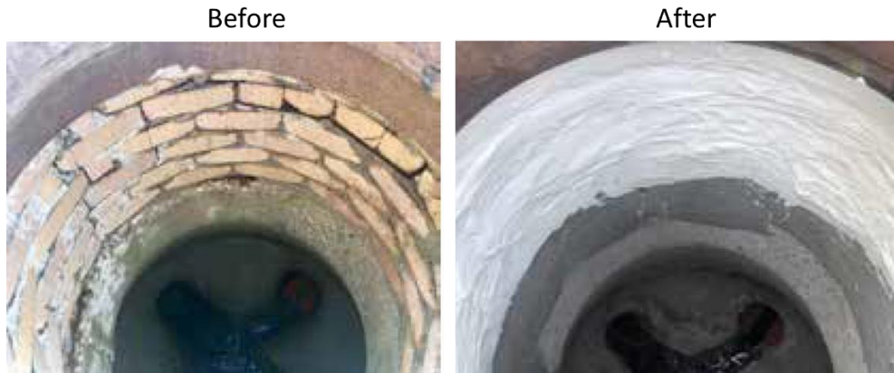
Figure 2.0-1 Typical Manhole Before and After Relining
