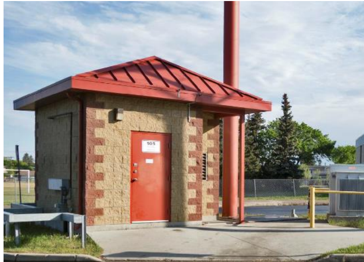
Figure 2.0-3 Duggan Pump Station
