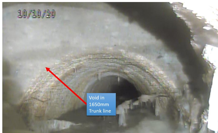
Figure 2.0-3 Void Inside 61 Avenue Trunk
