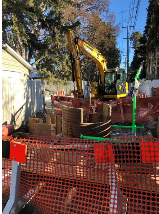
Figure 2.0-3 Typical Job Site for Deeper Mainline Replacement
