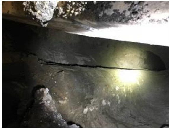
Figure 2.0-2 Severe Deterioration of 61 Avenue Trunk
