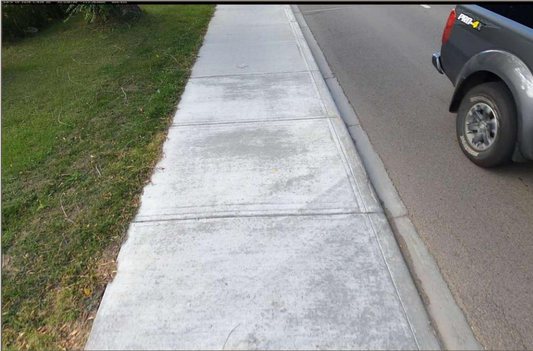
**Photo 4:** 111 Avenue, August 2020: Difference in concrete surface colour due to removal of curing compound.
