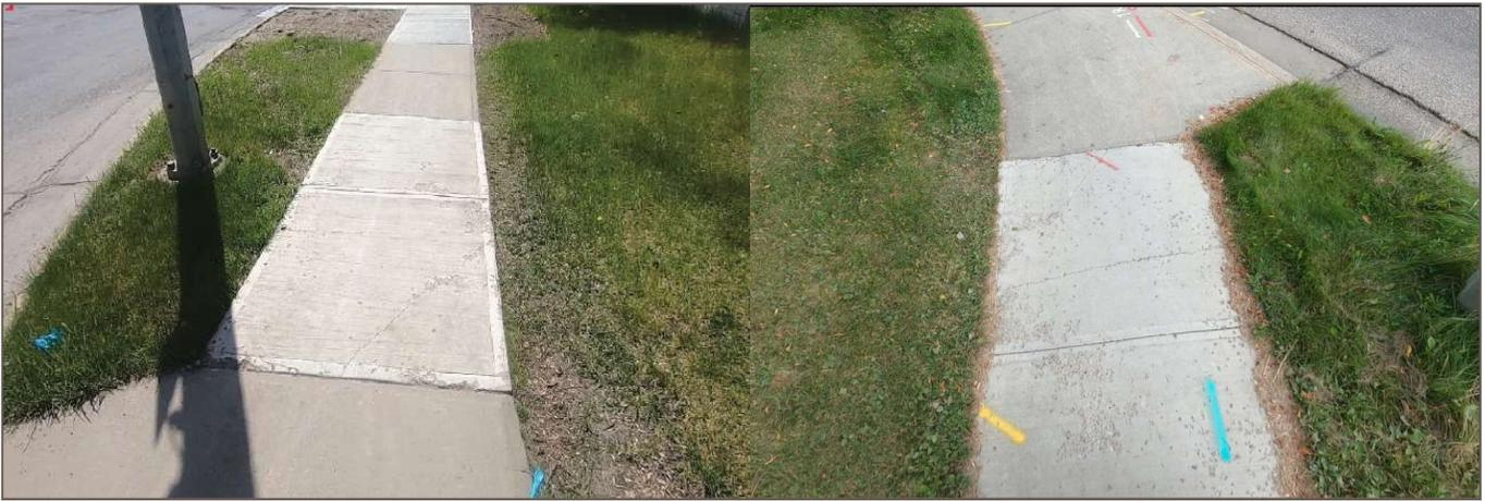
**Photo 9:** 178 Street: May 2019 photo on left, August 2020 photo on right. Severe scaling on panel likely construction related. Likely to be removed.
