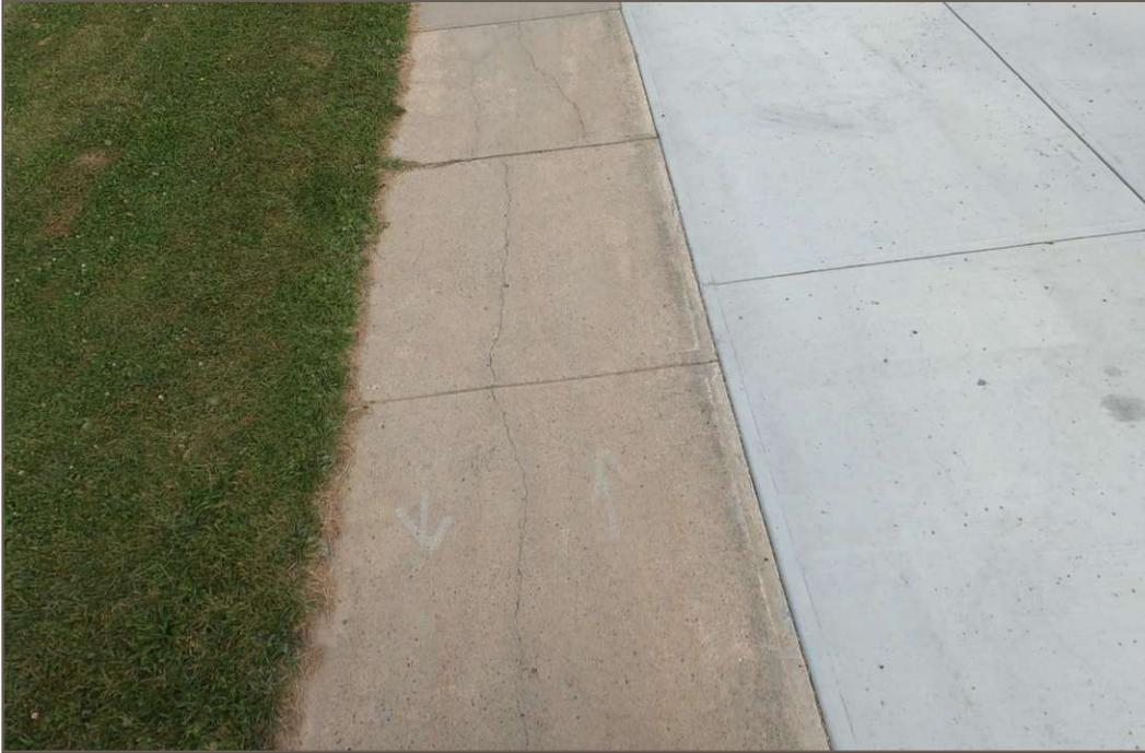
**Photo 10:** 178 Street, August 2020: Minor mortar flaking on concrete apron on right side of photo.
