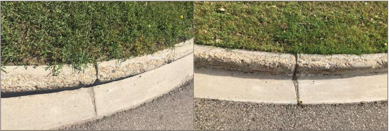
**Photo 11:** 50 Street and 106A Avenue: July 2019 photo on the left, September 2020 photo on the right. No visible increase in snowplow damage at rounded curb transition.
