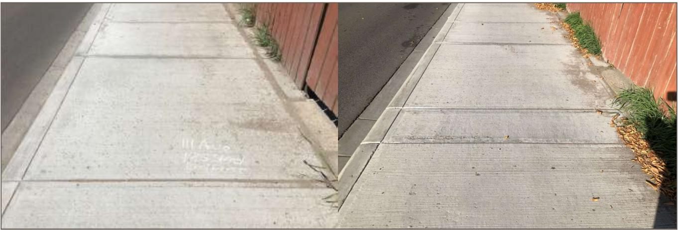
**Photo 2:** 111 Avenue: July 2019 photo on left, September 2020 photo on right. No noticeable change in mortar flaking volume.
