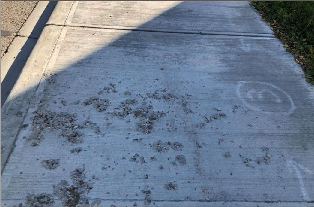
**Photo 6:** 111 Avenue, September 2020: One panel with severe scaling, likely to be removed.
