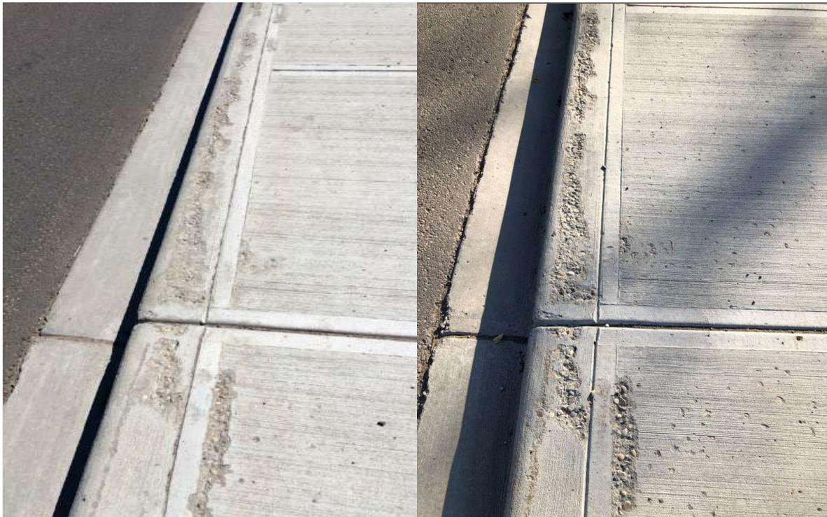
**Photo 3:** 111 Avenue: July 2019 photo on left, September 2020 photo on right. No noticeable difference in damage to volume of concrete removal by snow clearing equipment.
