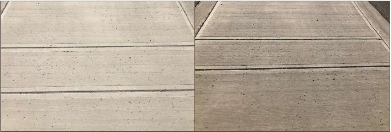
**Photo 12:** 50 Street and 101 Avenue: July 2019 photo on the left, September 2020 photo on the right. No visible increase in volume of mortar flaking.
