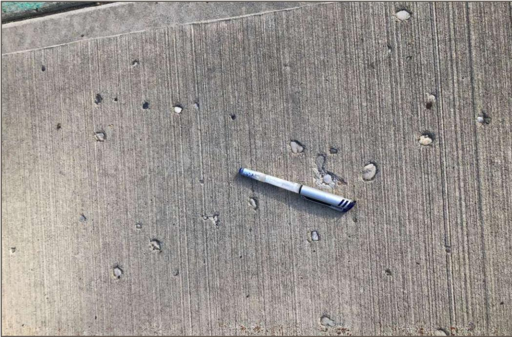
**Photo 1:** 122 Street near Fox Drive, September 2020: Mortar flaking on sidewalk surface caused by drying of surface above coarse aggregate.
