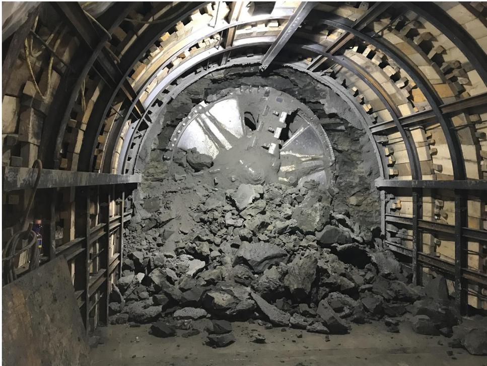
**Figure 1e – SESS SW4, Tunnel Boring Machine Breakthrough**
