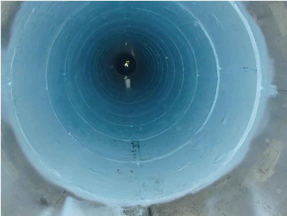
**Figure 1c – NEST NC2/NC3, Trunk with Epoxy Coating**
