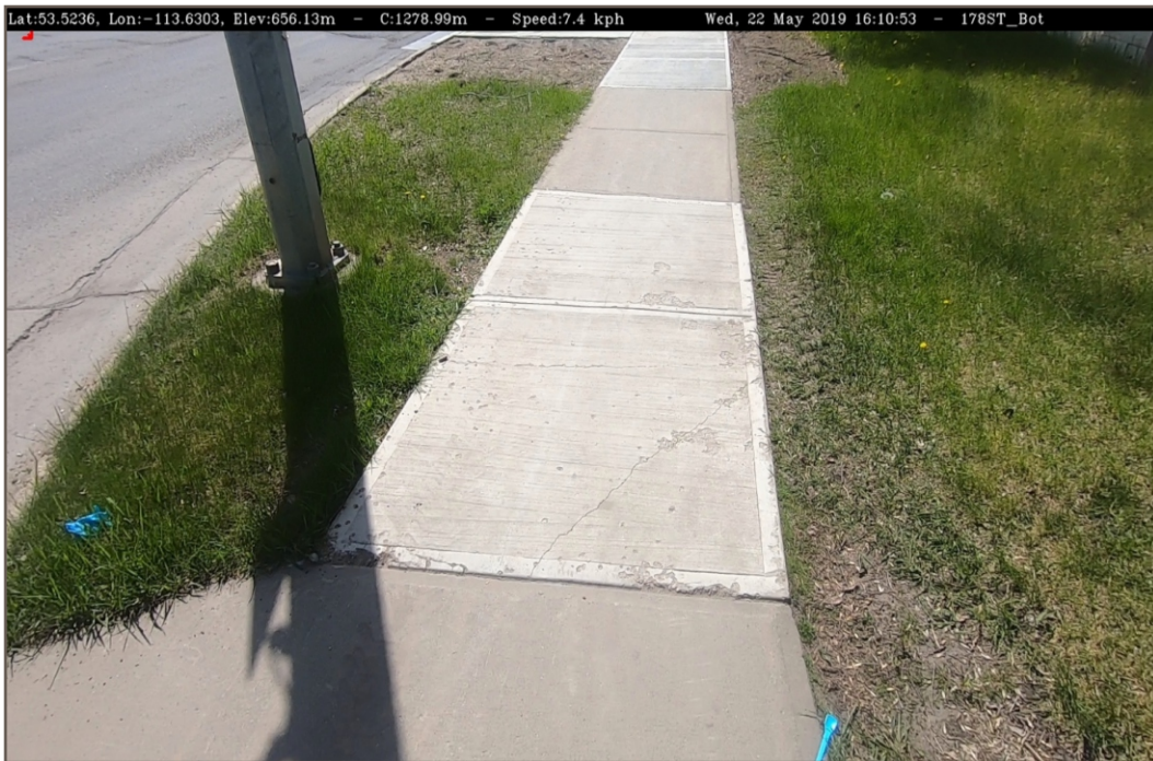
Photo 8: 178 Street. 2019 photo. Appears the two replacement concrete panels were poorly constructed. Newer concrete 2 panels up appear in good condition.
