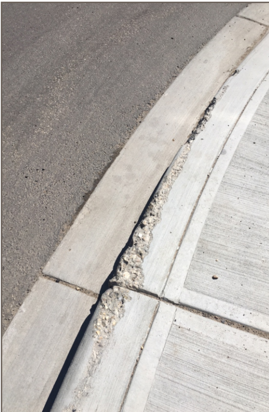
Photo 5: 111 Avenue. Photos obtained in 2019. Significant amount of damage to curb constructed in 2018.
