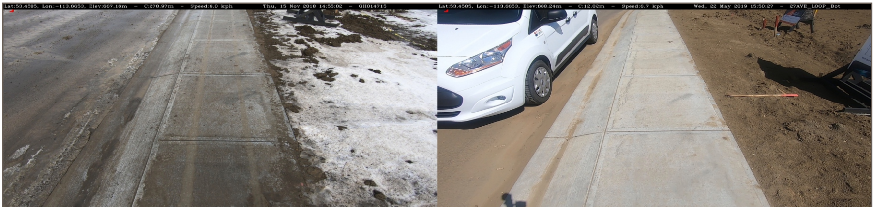
Photo 10: Uplands. 2018 photo on left, 2019 photo on right. Surface scuffing of the sidewalk near the back of curb is visible in spring 2019. Scuffing not present in fall 2018.
