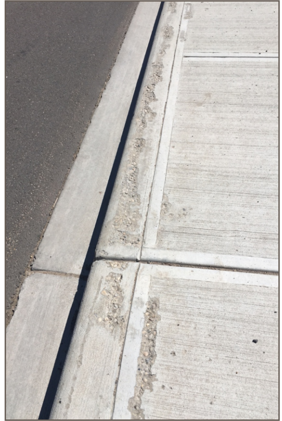
Photo 4: 111 Avenue. Photo obtained in 2019. Surface damage on surface of curb and sidewalk likely caused during snow removal.
