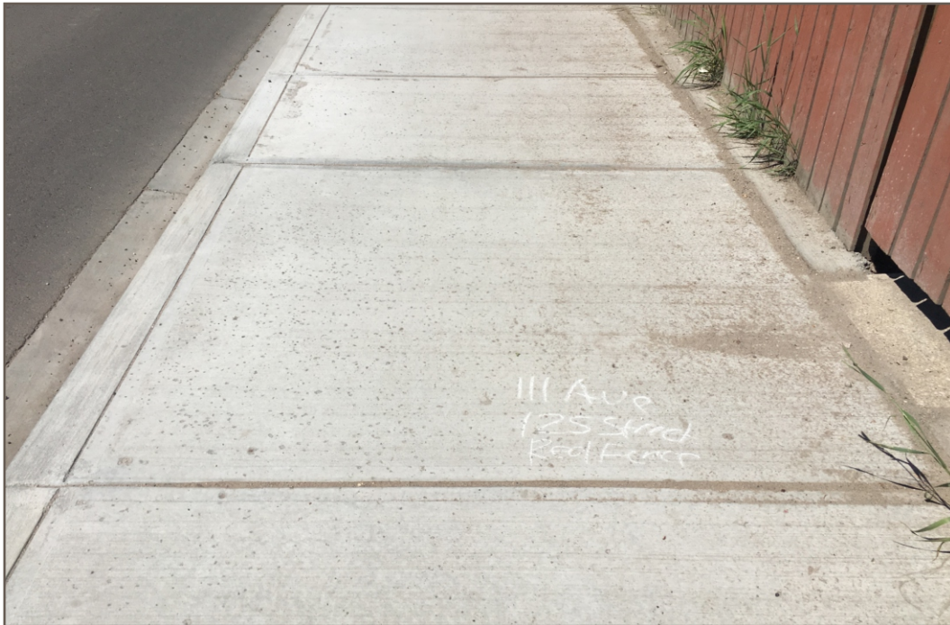
Photo 2: 111 Avenue and 125 Street. Photo obtained in spring of 2019. Concrete with mortar flaking on surface.
