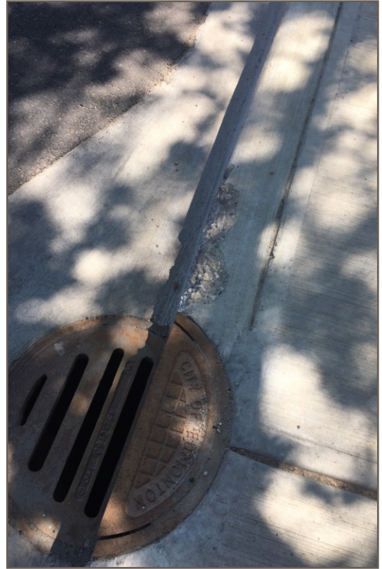
Photo 6: 111 Avenue. Photo obtained in 2019. Chipped concrete curb next to catch basin.
