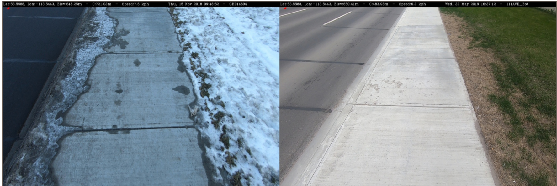
Photo 3: 111 Avenue. 2018 photo on left, 2019 photo on right. Spalling of concrete observed in 2019 image on right. Significant damage observed only on a single panel.
