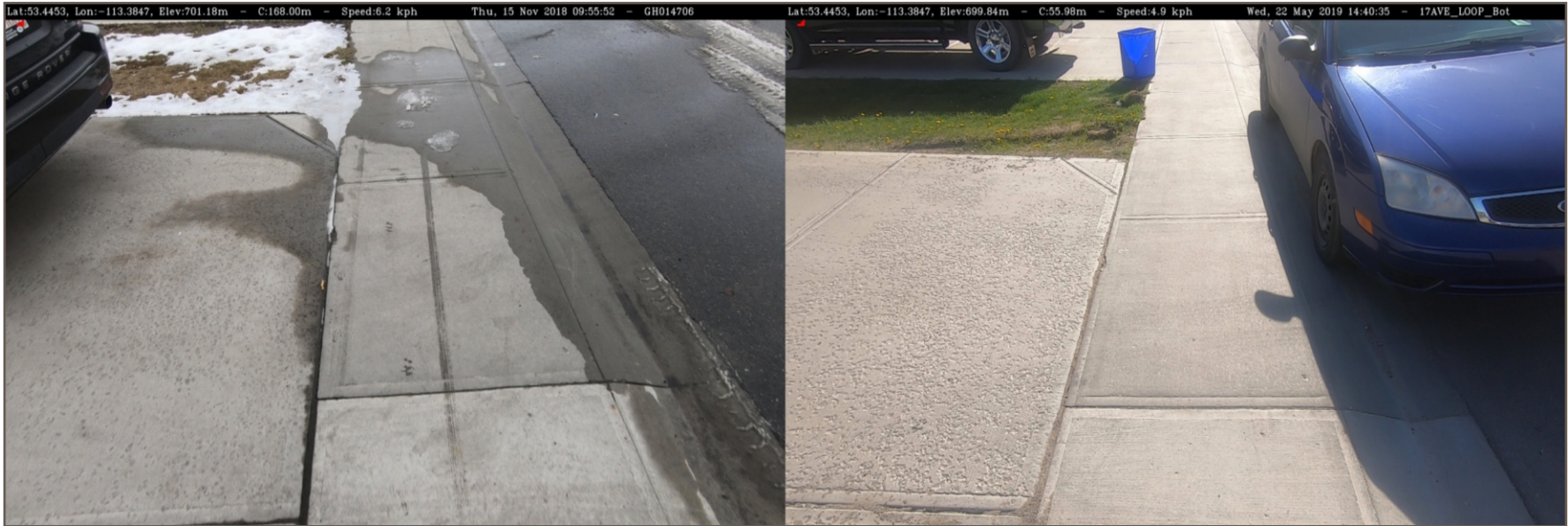
Photo 12: Laurel. 2018 photo on left, 2019 photo on right. Private driveway exhibiting significant damage while adjacent sidewalk is in good condition.
