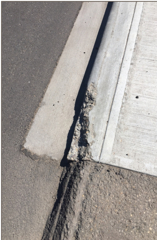
Photo 7: 111 Avenue. Photo obtained in 2019. Chipped concrete curb next to asphalt path.
