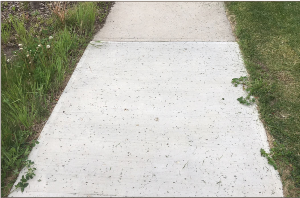
Photo 11: Laurel. 2019 photo. Concrete possibly damaged by chipping of ice from surface.
