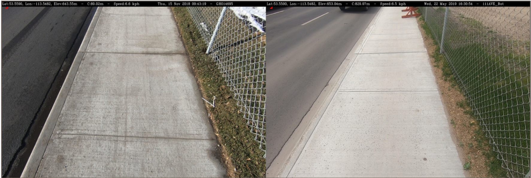
Photo 1: 111 Avenue. 2018 photo on left, 2019 photo on right. 2018 photo indicating little surface damage while in 2019 some mortar flaking is visible within ~1 m of the curb.
