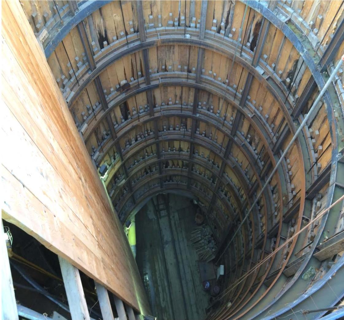
**Figure 1h: SESS Stage SW4- 16'-6" diameter Working Shaft, depth of 18.0 m below ground elevation**
