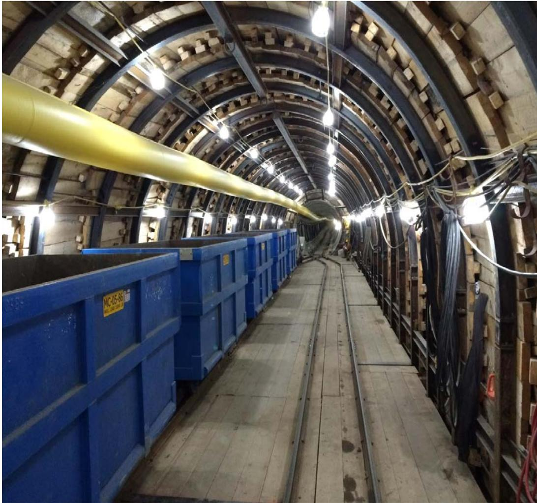
**Figure 1e: SESS Stage SW4- Tunnel undercut, total length of 32 m, dirt cars on rail switch set-up**
