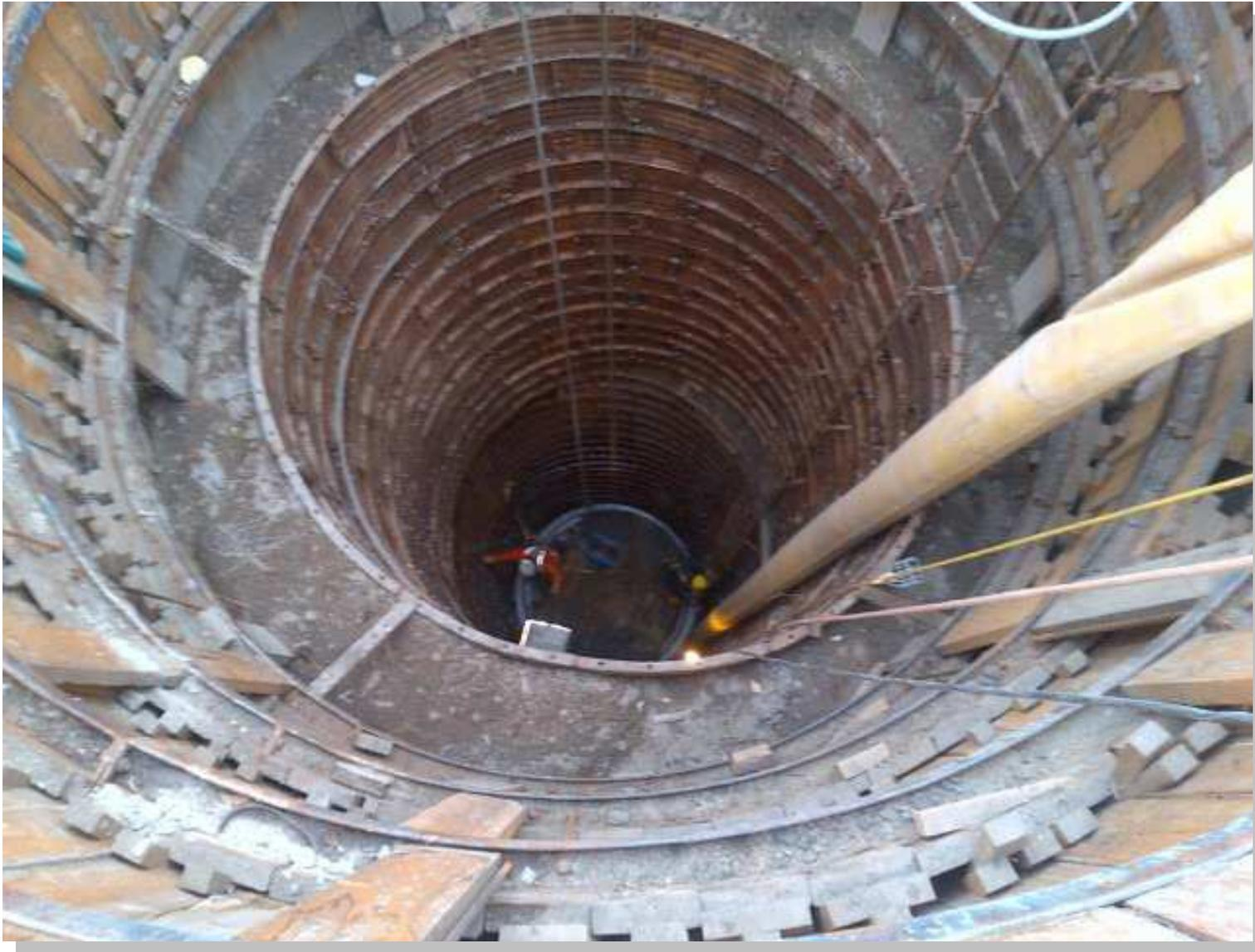
**Figure 1d. NEST NL2/NL3/N1 – Construction of Access Manhole**
