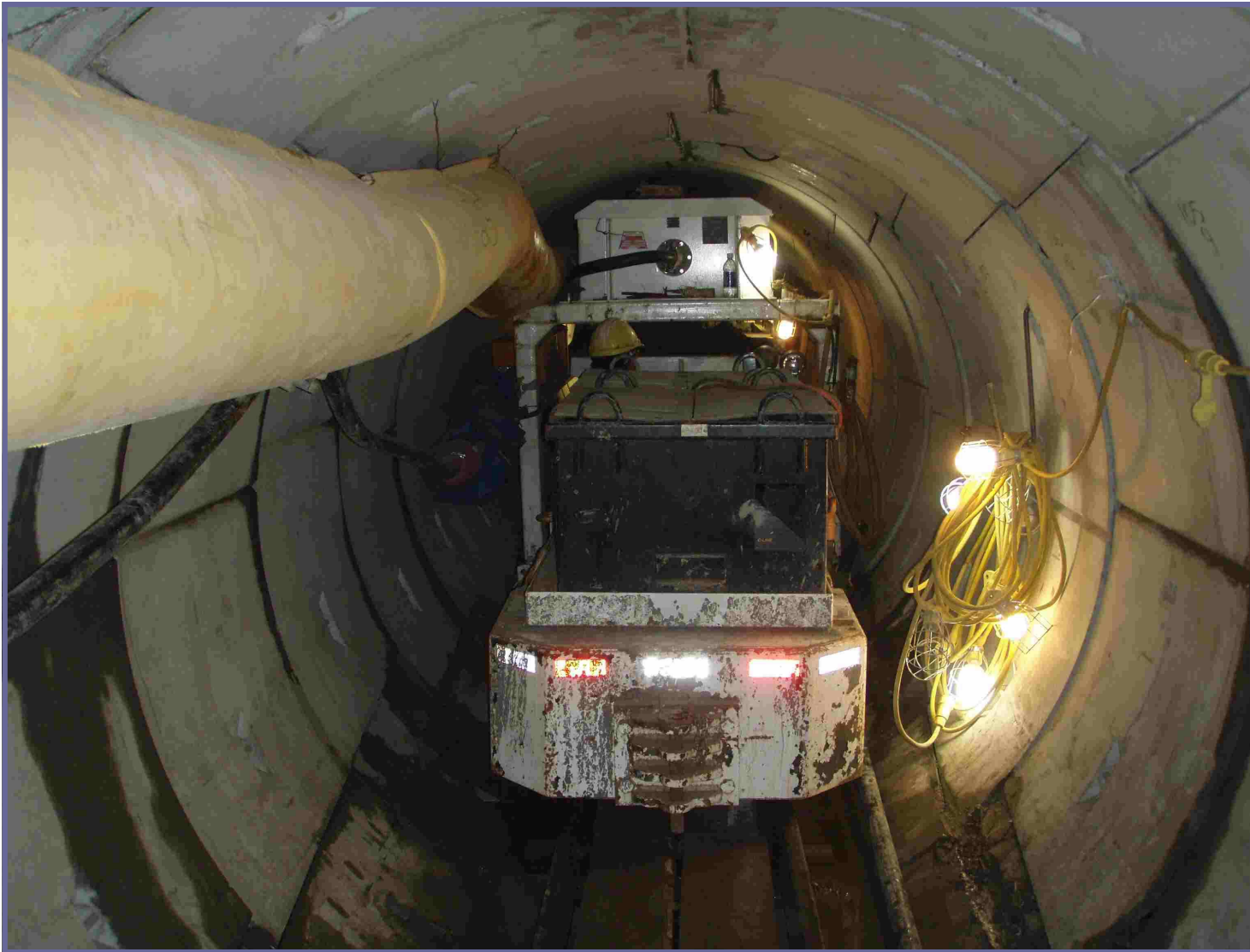
Figure 1c. SESS Stage SA1b: Tunnel liner in place
