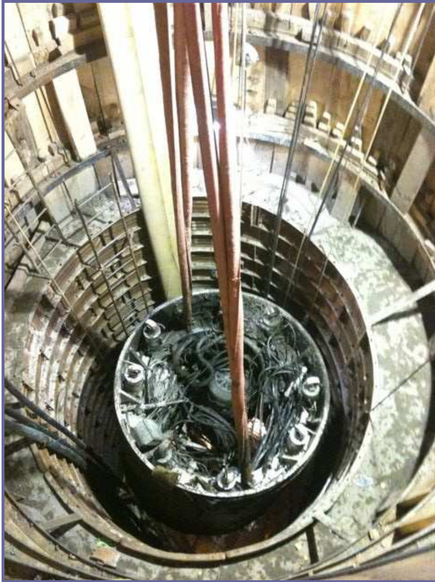
Figure 1b. NEST Stages NL1/NL3/N1: Mole removal at the 75 Street shaft
