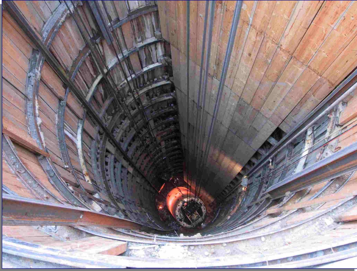
**Figure 1b. SESS Stage SW2-3: Mole lowered into shaft and undercut**
