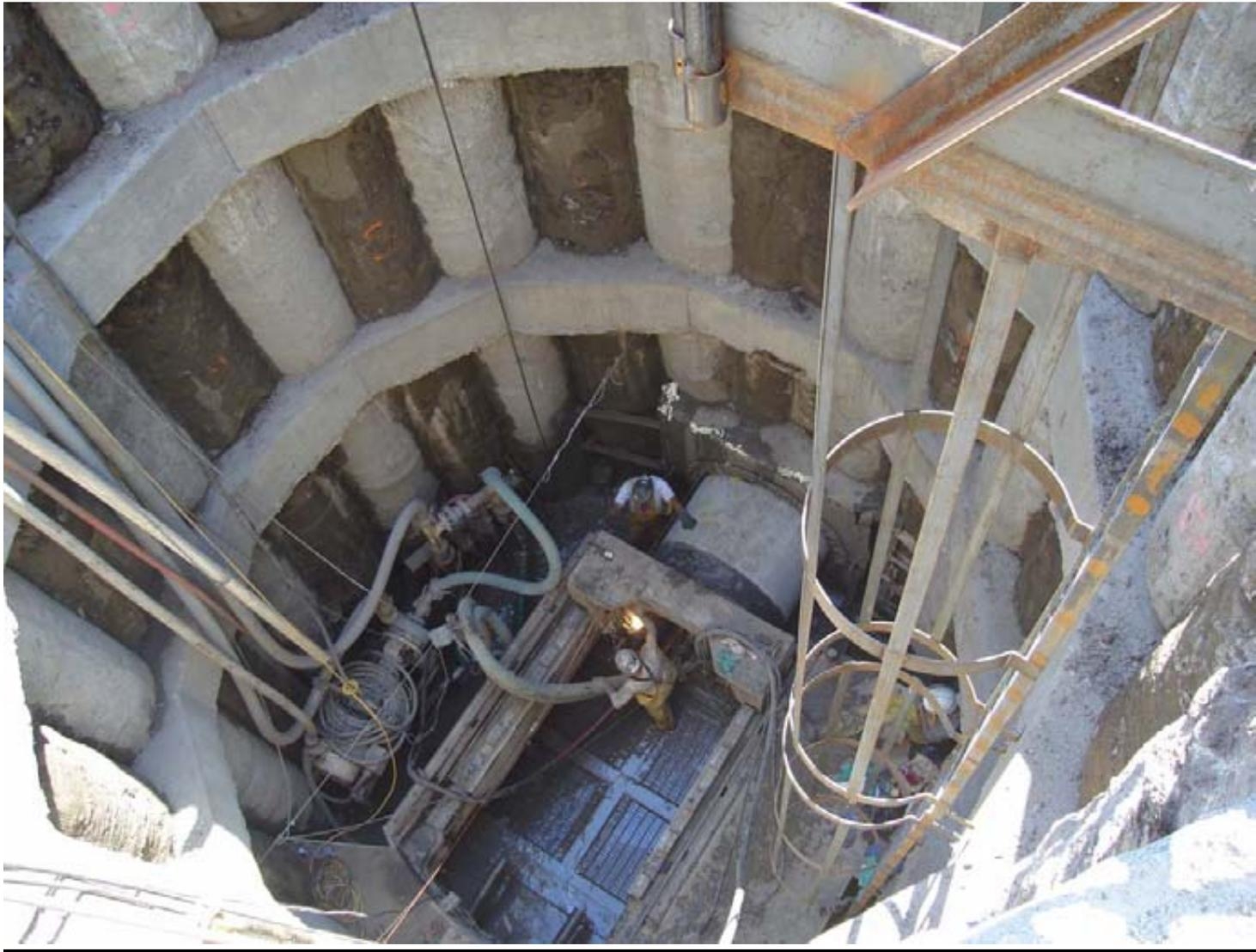
Figure 1(d)-WESS (W1) – Microtunnelling in Progress
