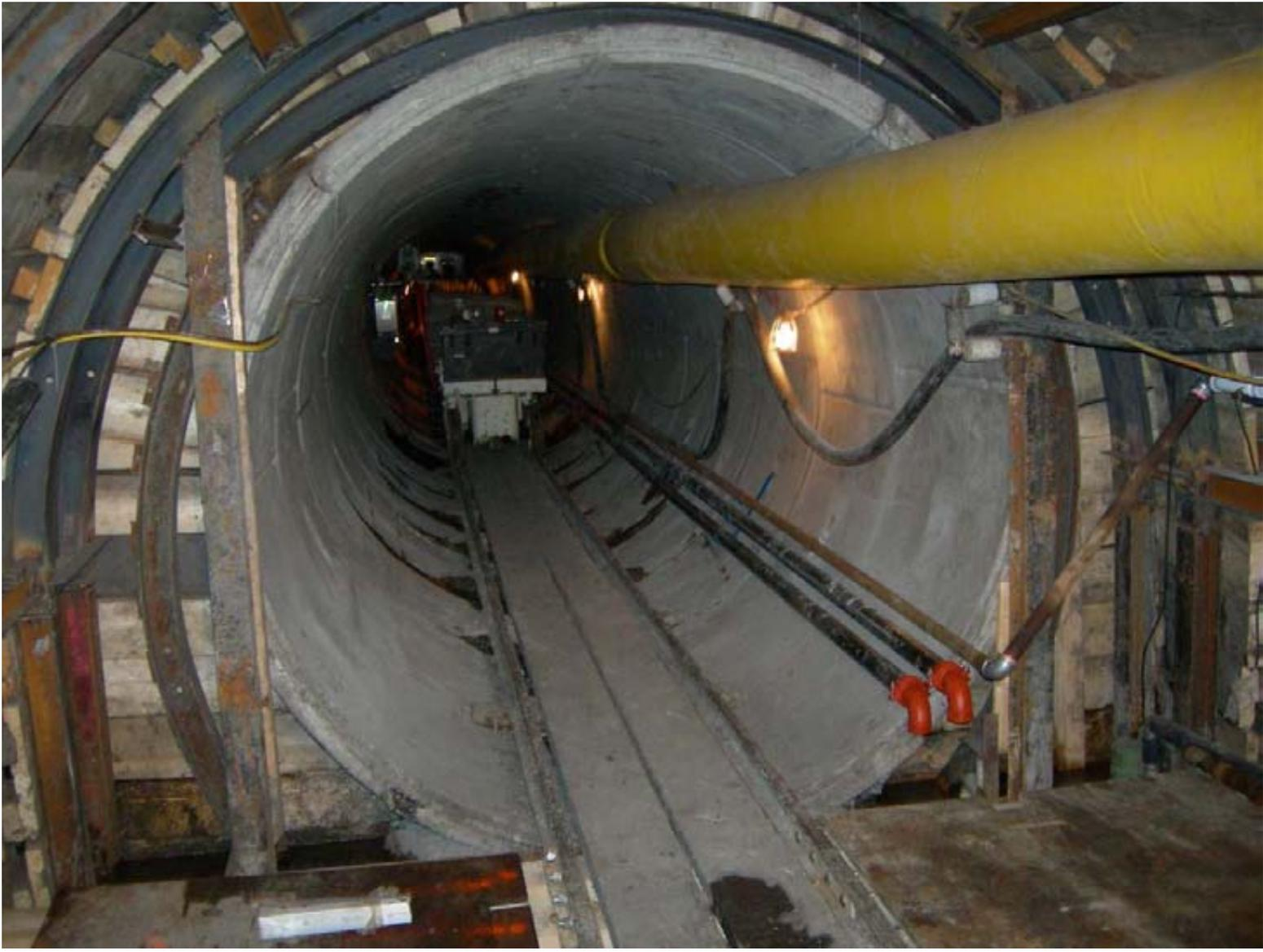
Figure 1(C) SESS (SW2/3) – Tunnel Finished with Concrete Liners
