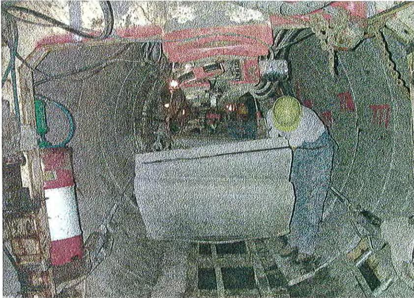
A member of the NC1 tunneling crew guides tunnel sections to the back of the TBM for installation. Four precast concrete sections form a 1.0m length of tunnel. The completed tunnel can be seen in the background.
