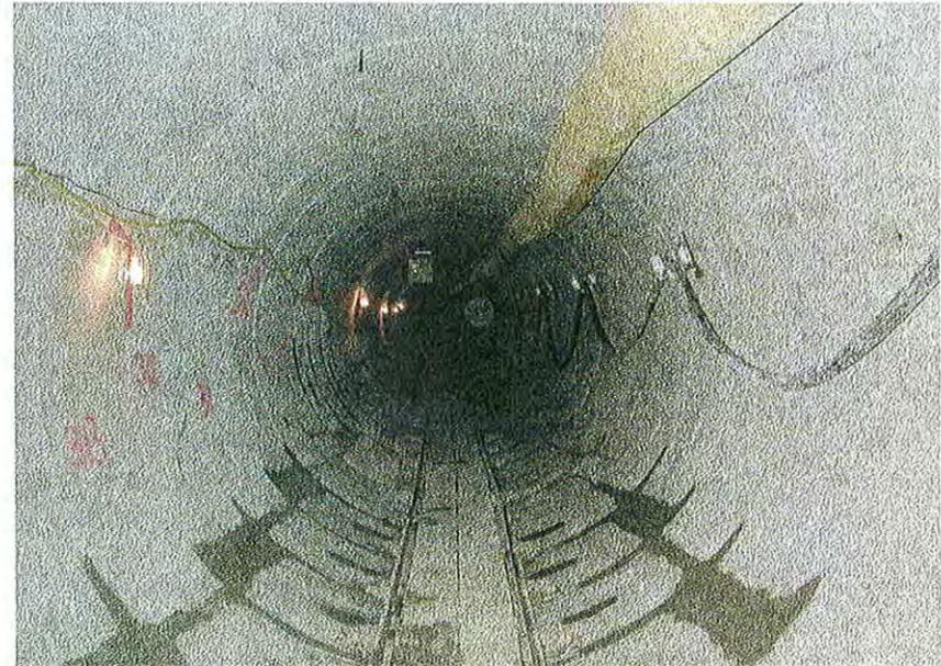
Completed section of the NC1 tunnel. Piping for ventilation and power cables can be seen on the top right and the right side of the picture. The railway track at the bottom of the picture allows rail cars to bring construction material in and take tunneling spoil out through the construction access shaft.
