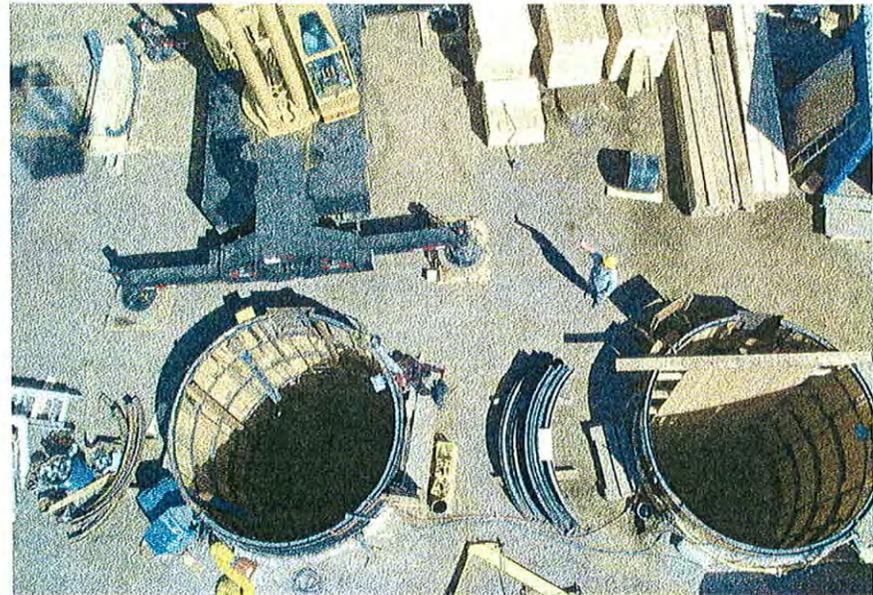
Drop shafts for NC1 located at NW corner of 153 Avenue & Castle Downs Road (113A Street). This is the location of the pump station. The right (east) shaft is the dry well, where the pumps will be located. The left shaft is the construction access shaft. After construction, it will be the wet well, where sewage is received from the tunnel to await pumping.
