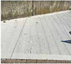
1 SAW CUT BROOM FINISH CONCRETE
