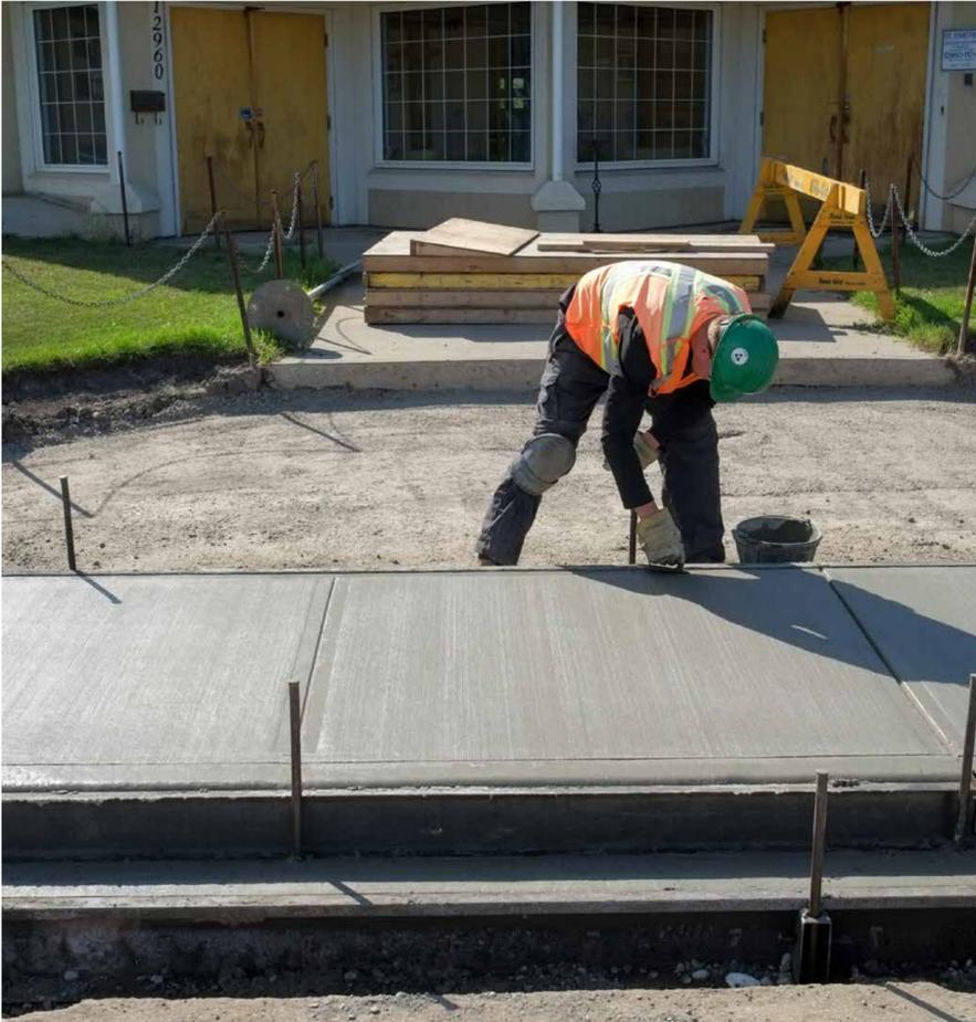
If a sidewalk is machine poured, a stringline is used to set grades as it pours the concrete.
