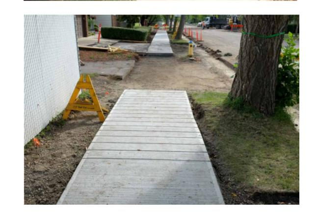
An area around each tree is maintained during construction to protect it and its roots.
