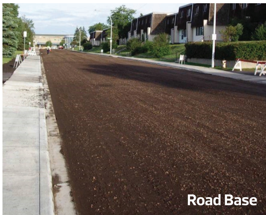
Pulverizing and Mixing the Road
