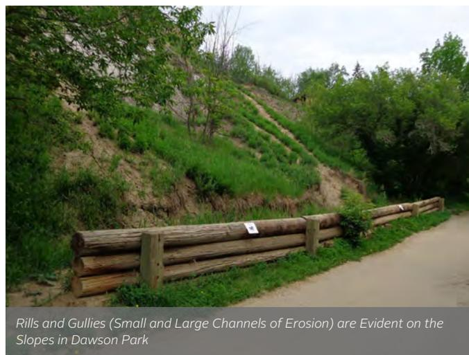
Rills and Gullies (Small and Large Channels of Erosion) are Evident on the Slopes in Dawson Park
