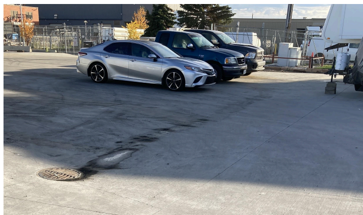
Figure 10 - Example of Concrete Pad with Swale
