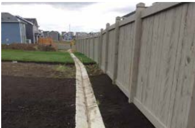
Figure 15 - Major concrete drainage swale easement
