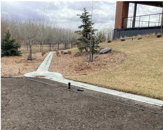
Figure 8 - Example of Internal Concrete Swale
