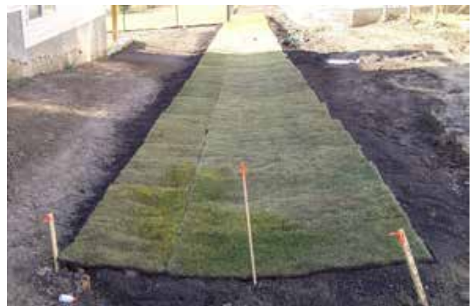
Figure 16 - Major grass drainage swale easement
