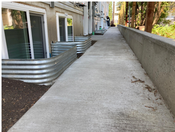
Figure 11 - Concrete Retaining Wall
