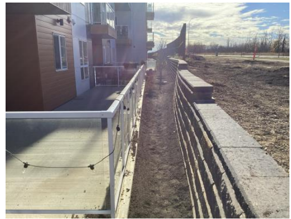
Figure 12 - Stone Retaining Wall
