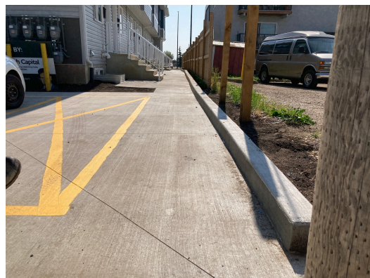
Figure 13 - Concrete Curb as Retaining Wall
