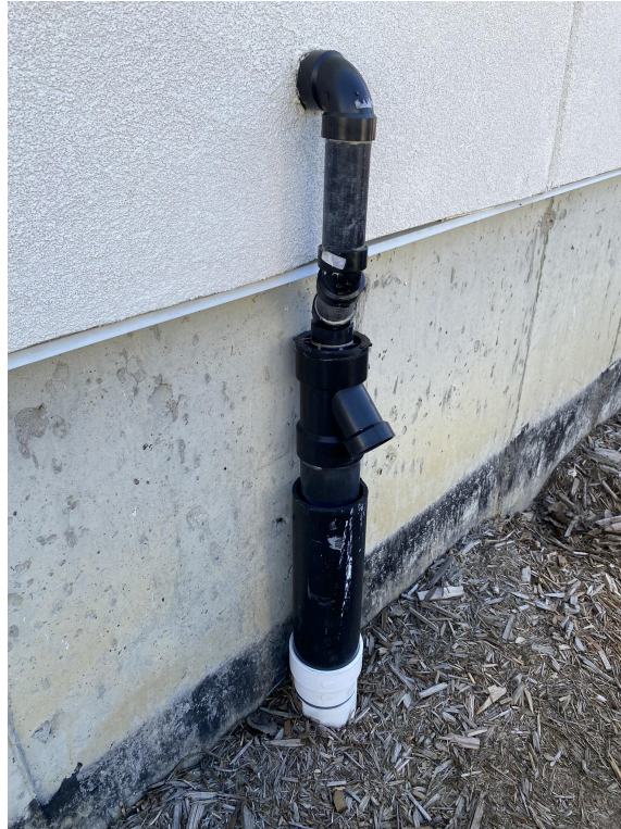
Figure 18 - Sump discharge detail
