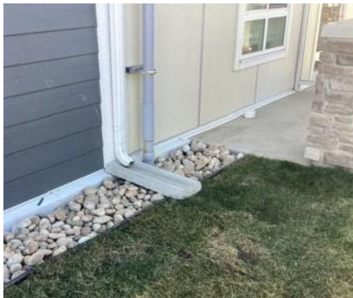
Figure 17 - Splash pad under downspout
