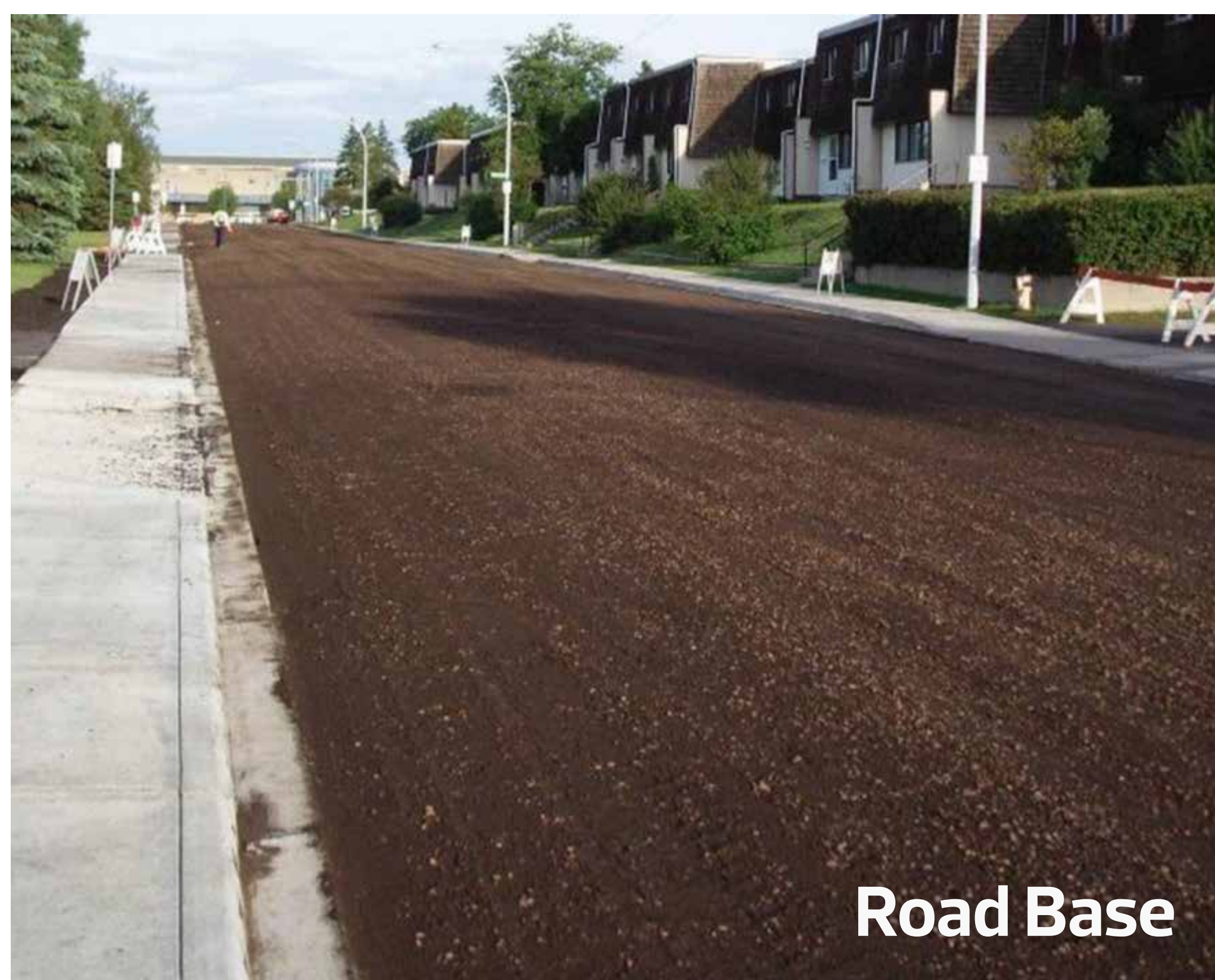
Pulverizing and Mixing the Road
