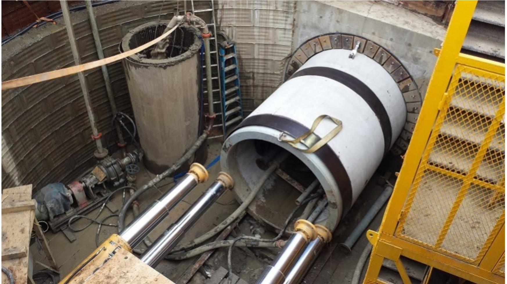
**Figure 1a: SESS Stage SA1a- Pipe Jacking station**
