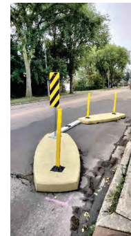
Adaptable curb extension on 102 Street and 82 Avenue, as part of the Ritchie Street Lab.
