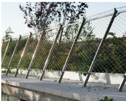
GALVANIZED HANDRAILS WITH MESH INFILL
