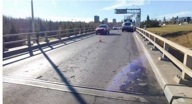
*Scona Road Bridge (B065) Deteriorated Concrete Bridge Pavement*
