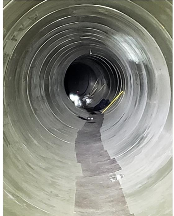
Figure 1c - SESS SW4, Completed Tunnel with Liner
