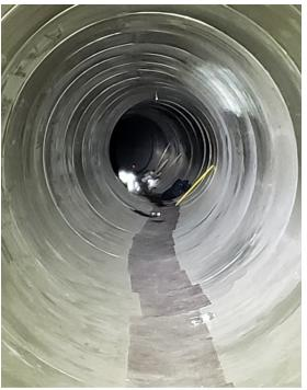
Figure 1c - SESS SW4, Completed Tunnel with Liner
