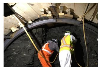
Figure 1b - NEST NC2/NC3, Undercut Excavation
