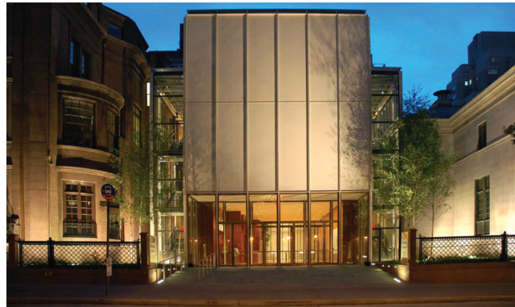
RESPECT IN CONTRAST: AN ARCHITECTURAL ADDITION STANDS NEAR A HISTORIC BUILDING, SET BACK FROM THE STREET, PRESERVING THE CHARM AND COEXISTING HARMONIOUSLY IMAGE MORGAN LIBRARY, NYC, NY. SOURCE RENZO PIANO BUILDING WORKSHOP
