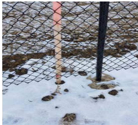
Large gaps - ensure that a 50mm gap from top of final grade to bottom of fence is achieved, or properly surveyed for documentation and clarity.
