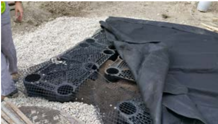
Soil Cell Installation
