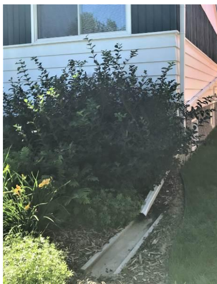
Photo 4: Roof Leader to Splash Pad Inlet
